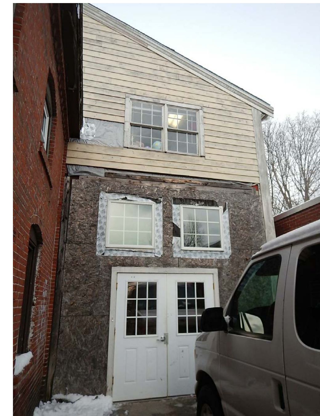
WEST FACADE OF WOOD-CLAD BUILDING
