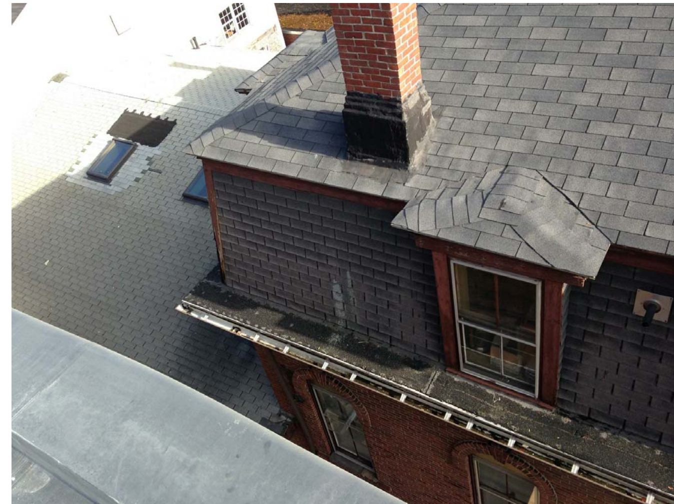
MANSARD ROOF & THIRD FLOOR WINDOWS
