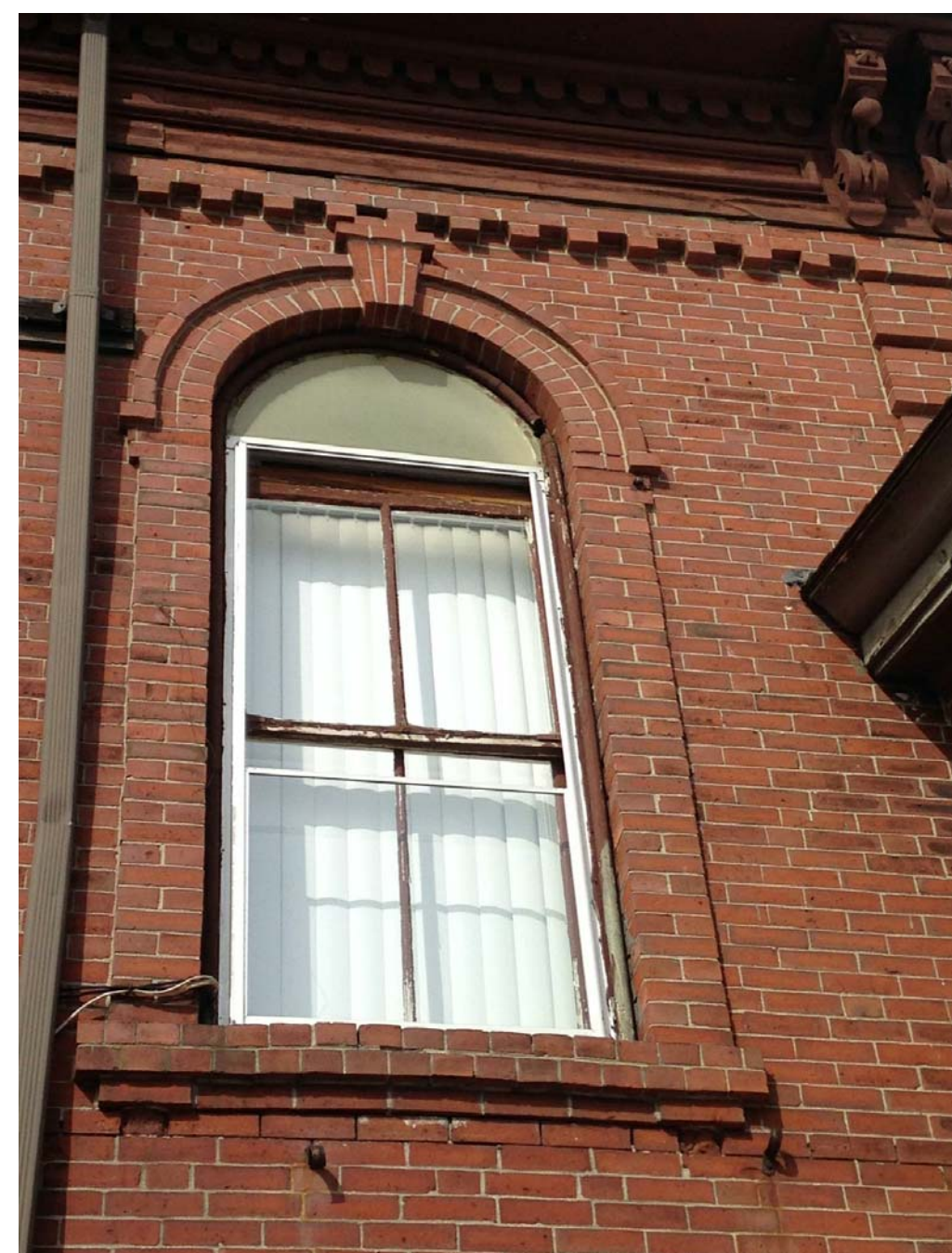
SECOND FLOOR ARCHED WINDOW
