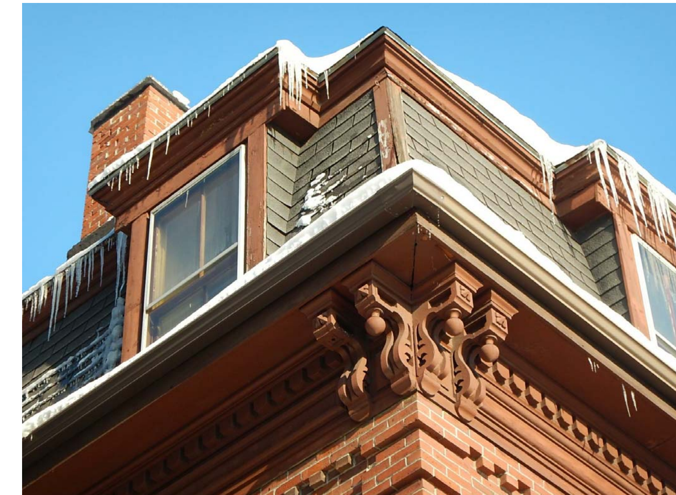
MANSARD ROOF & CORNICE DETAIL AT CORNER
