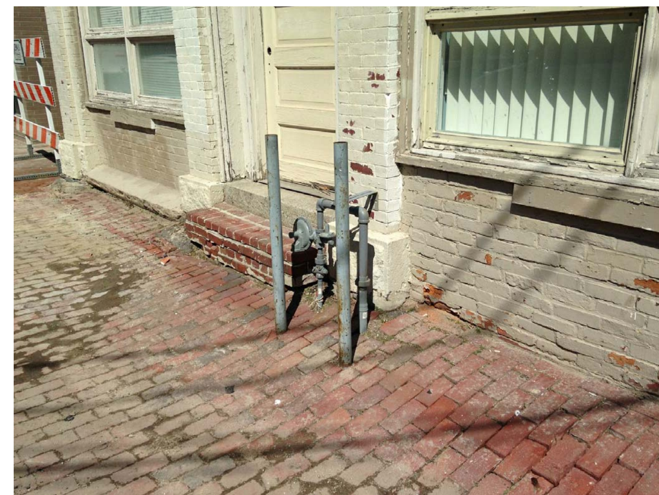
FRONT FACADE AT STREET LEVEL
