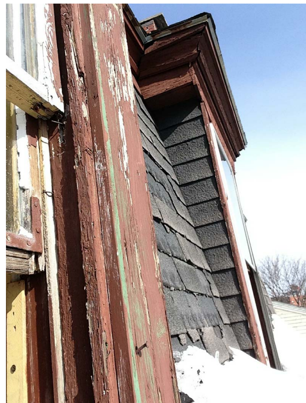
MANSARD ROOF & THIRD FLOOR WINDOWS
