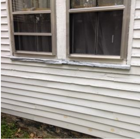
West (Rear) Face of Building Window Sills to be Replaced
