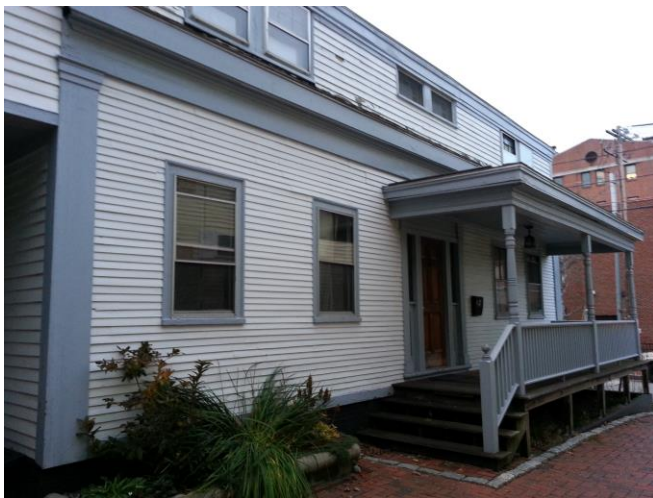
South Face of Residence
