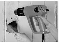
There work places will eliminate dust, but some renovation methods make less dust than others. Contractors may choose to use various methods to minimize dust generation, including using water to mist areas before sanding or scraping; scoring paint before separating components; and prying and pulling apart components instead of breaking them.
