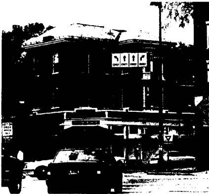
182 existing conditions from state street
