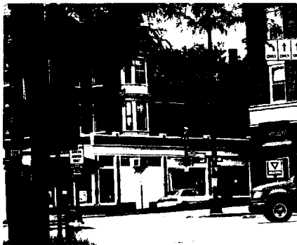
182 existing conditions from state street
