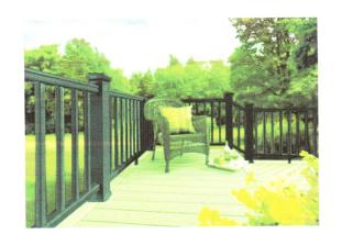
posts in this photo are 6x6 - ours would be 4x4 With Smaller ballusters closer together to meet code.
