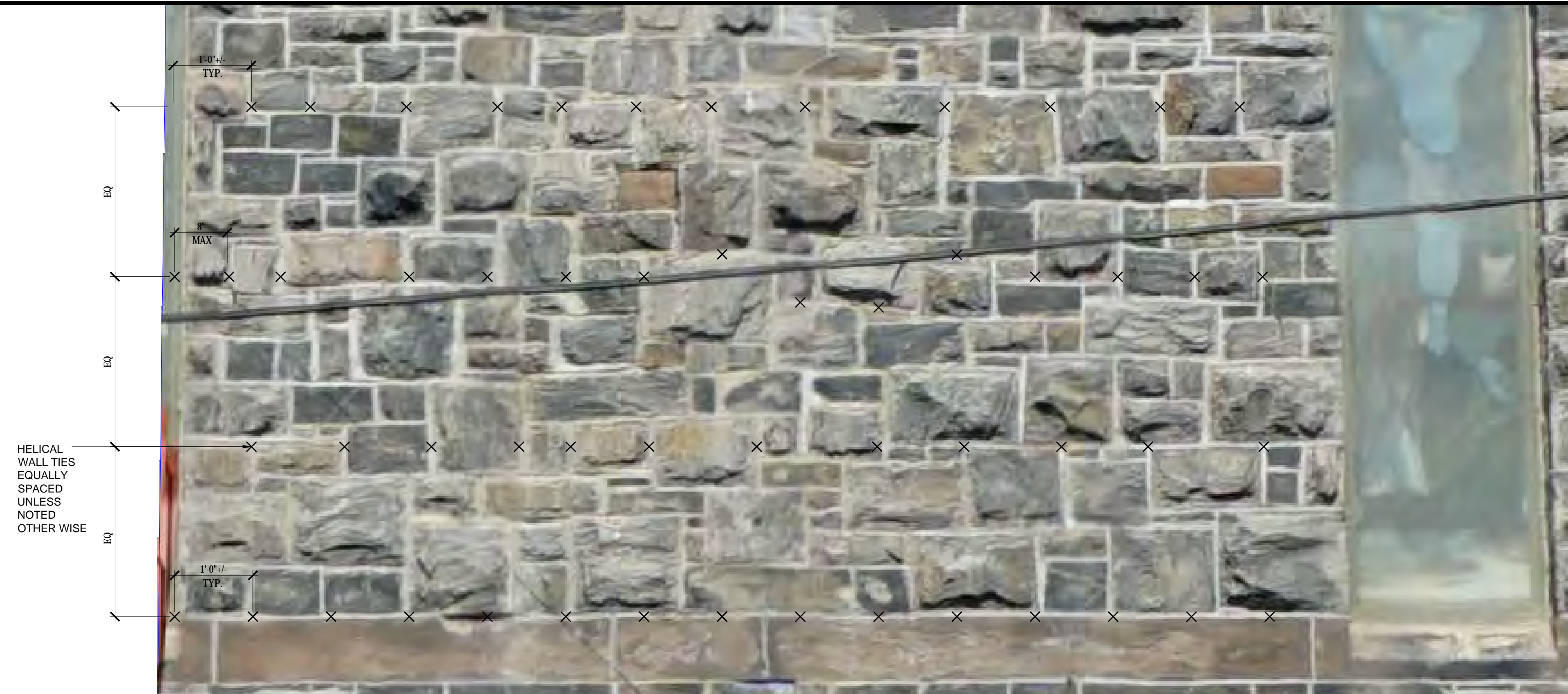
3 HELICAL WALL TIE PATTERN
