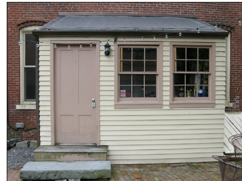
THE SHED ON THE BACK END OF THE HOUSE, BUILT IN 1992, THE RENOVATION OF WHICH IS THE SCOPE OF WORK OF THIS PROJECT. THE SHED ALSO SERVES AS THE ENTRY TO THE HOUSE FROM THE PARKING SPOTS OUTSIDE THE FENCE.
