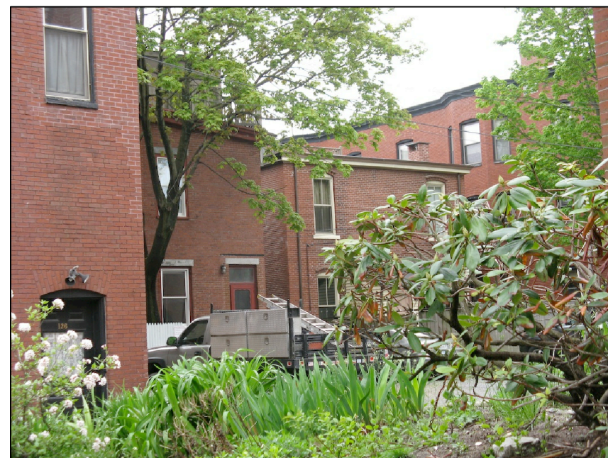
THE BACK OF THE HOUSE AS SEEN FROM THE PARK STREET SIDEWALK IN SUMMER
