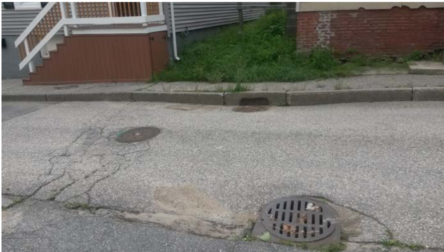
Existing Catch Basin
