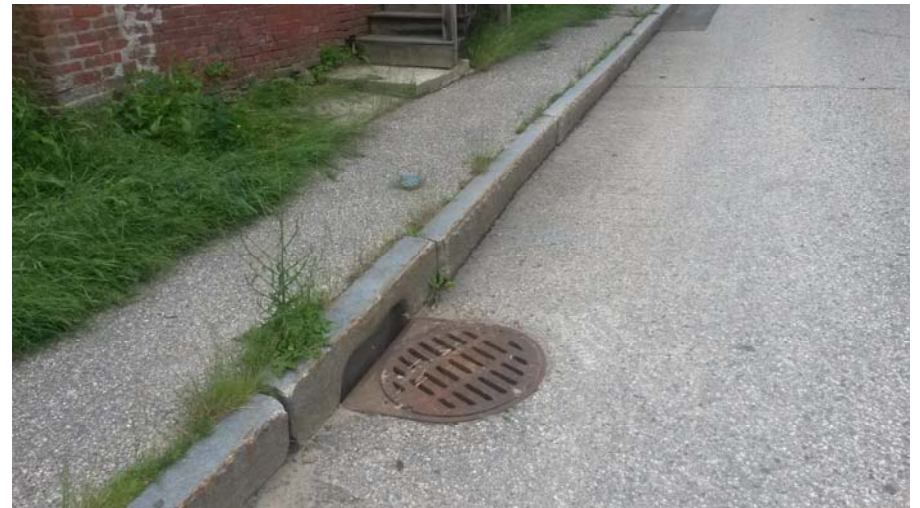
Existing Catch Basin
