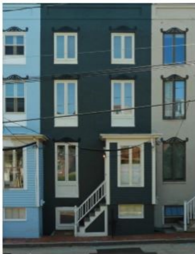
4 Stratton Place – Current Casement Windows
