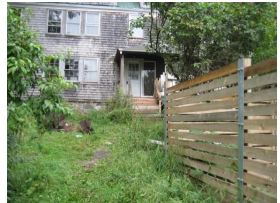
Existing building on the site
