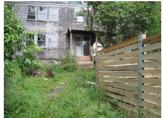
Existing building on the site
