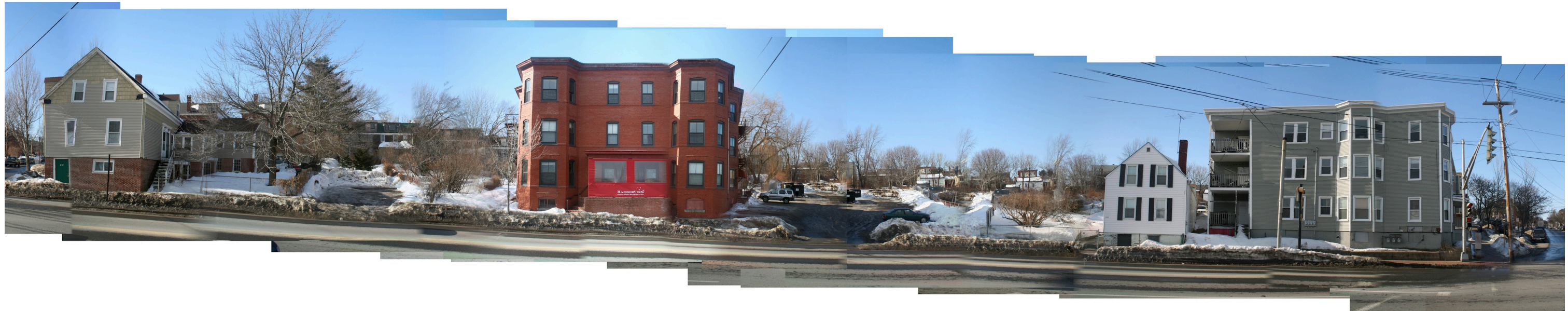
① VIEW FROM YORK ST: STREET FACADE
