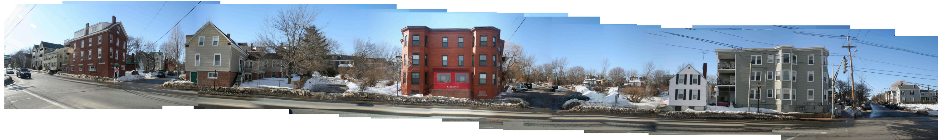
② VIEW FROM YORK ST: STREET FACADE
