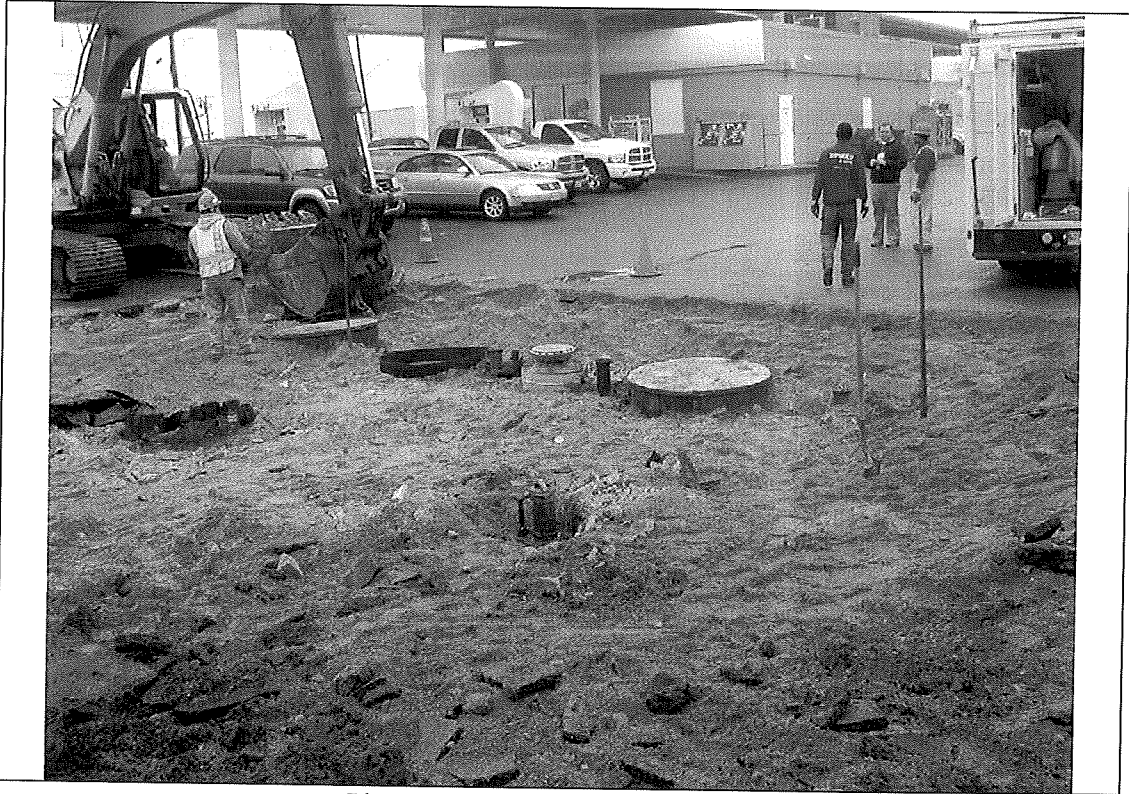
Photograph 1: Sumps facing south
