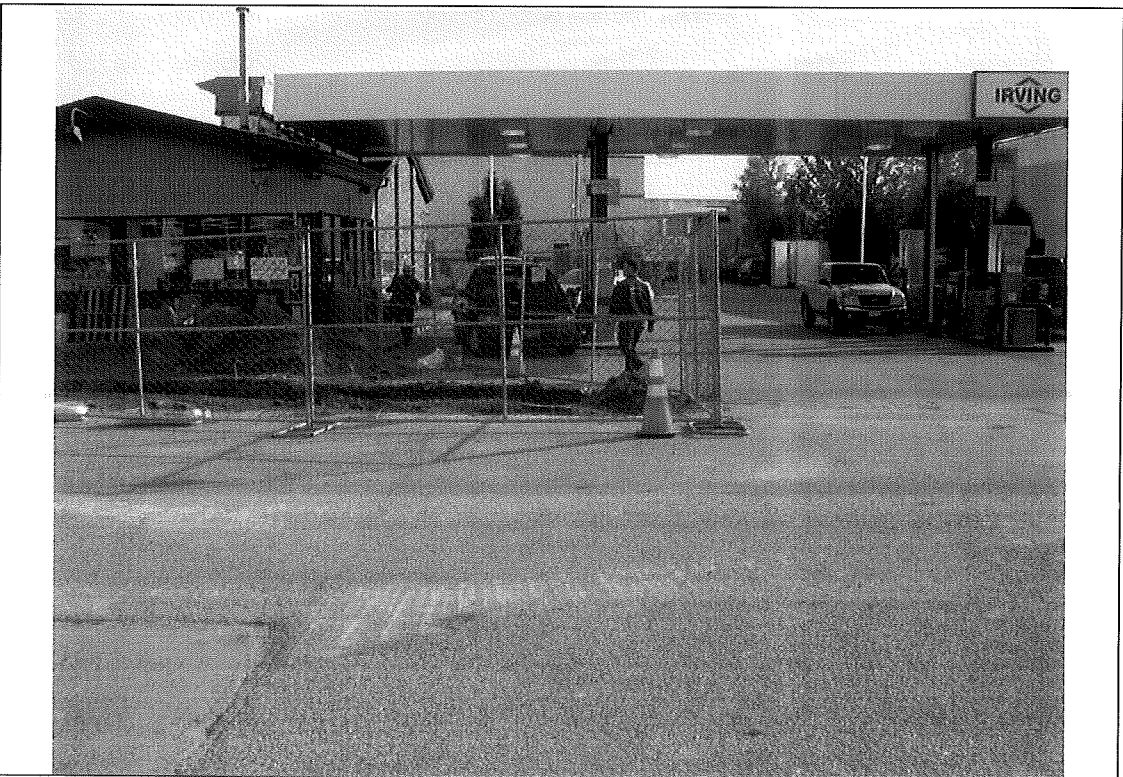
Photograph 2: Rear Canopy, facing south
