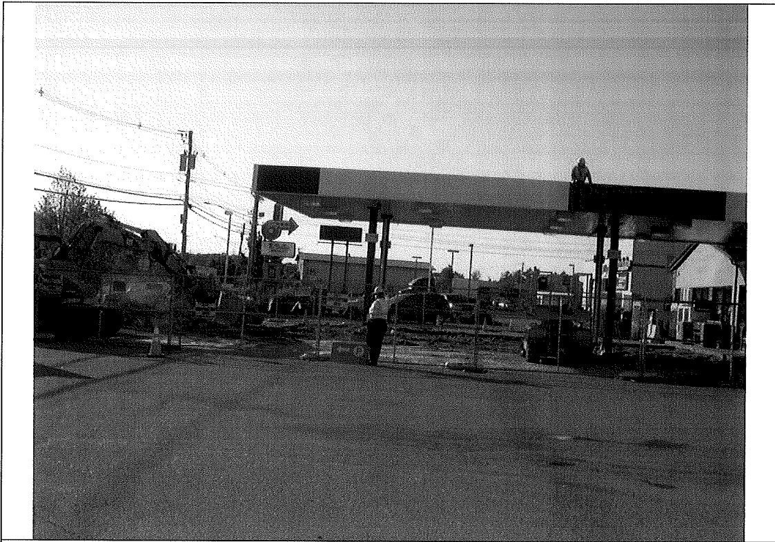
Photograph 1: Front Canopy, facing south
