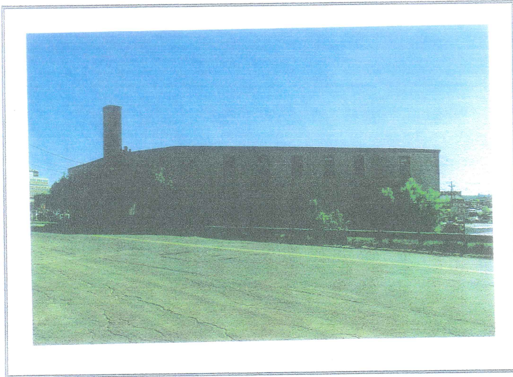
1) Easterly view of subject from York Street
