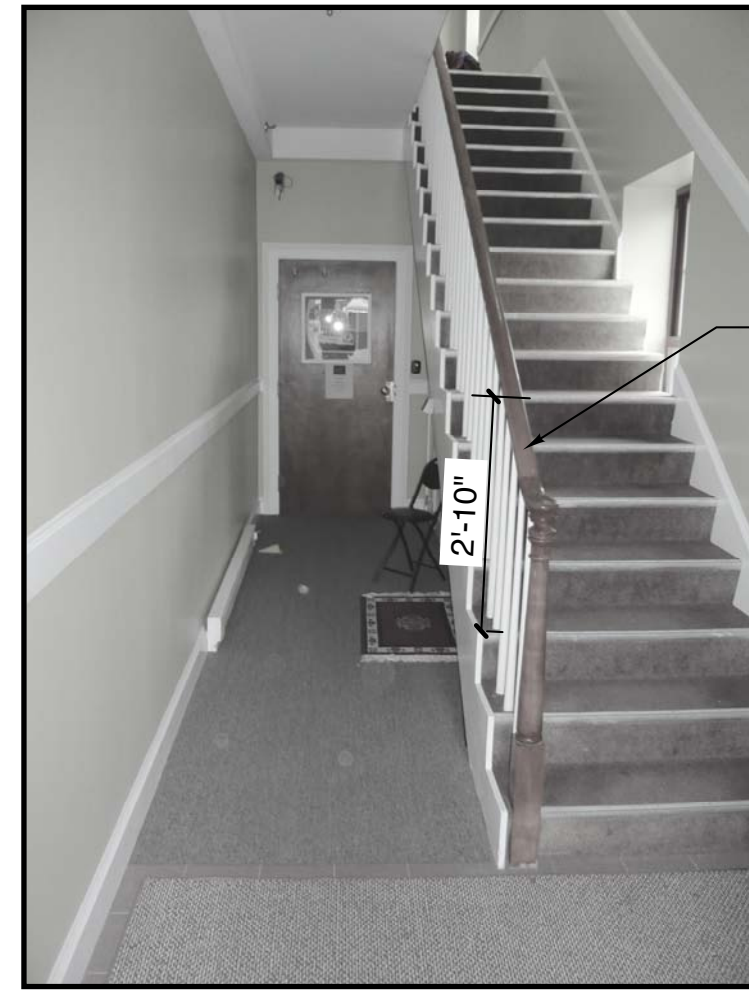
EXISTING WEST STAIR
