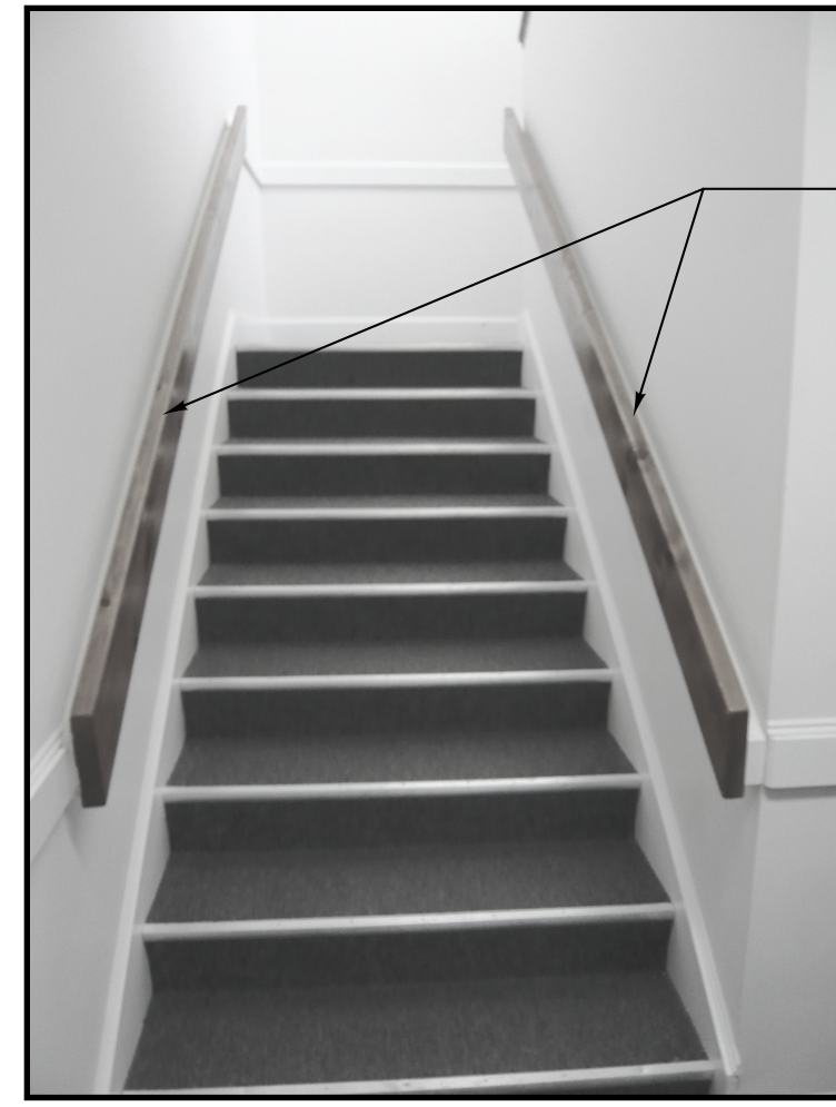
EXISTING EAST STAIR
