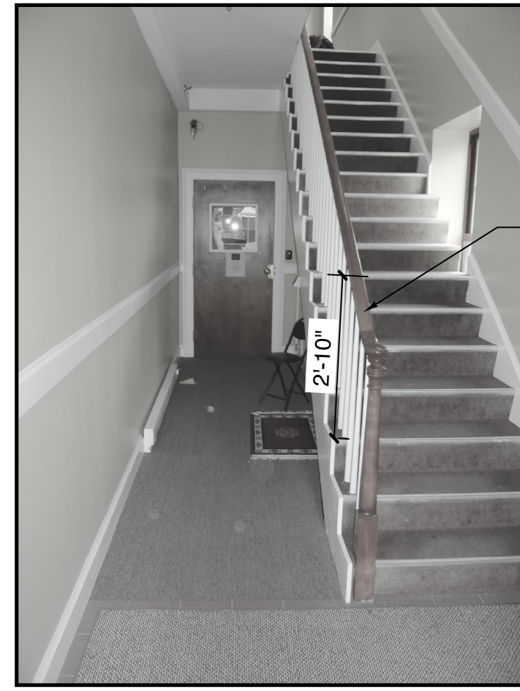
EXISTING WEST STAIR
