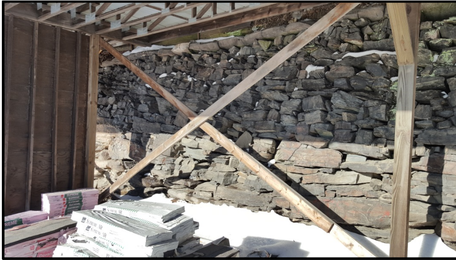
Figure 1: Existing rock retaining wall
