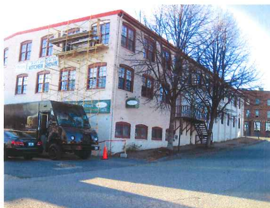
Location for Baxter Academy on opposite side of Maple St
