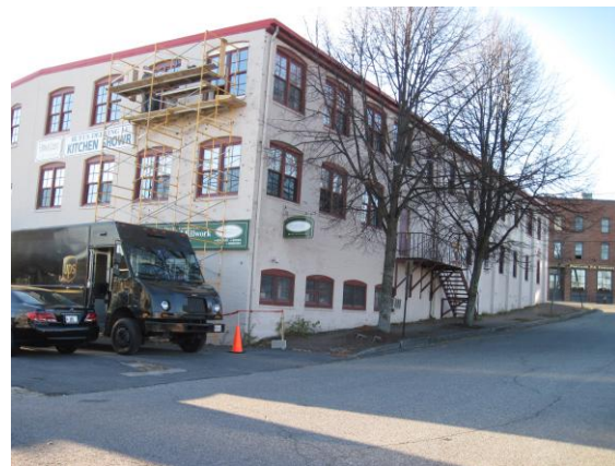
Location for Baxter Academy on opposite side of Maple St
