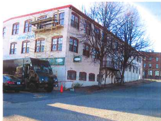
Location for Baxter Academy (high school) on opposite side of Maple St
