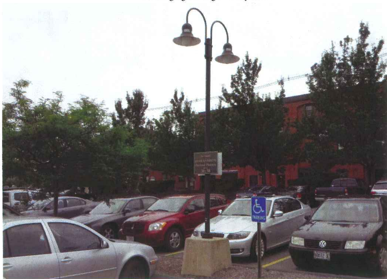
Existing light within upper parking lot
