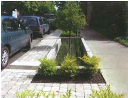
Depending on how intense a particular storm is, runoff will continue its downhill "dance" from planter to planter until all of the stormwater planters are at capacity. Once exceeding capacity, the water exits the last stormwater planter and enters the storm sewer.
