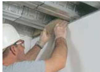
Full coverage pre-cut flute configuration leaves no gaps or voids.
