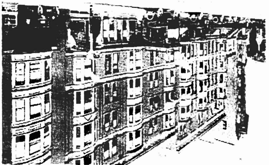
REAR VIEW OF THE BUILDING
