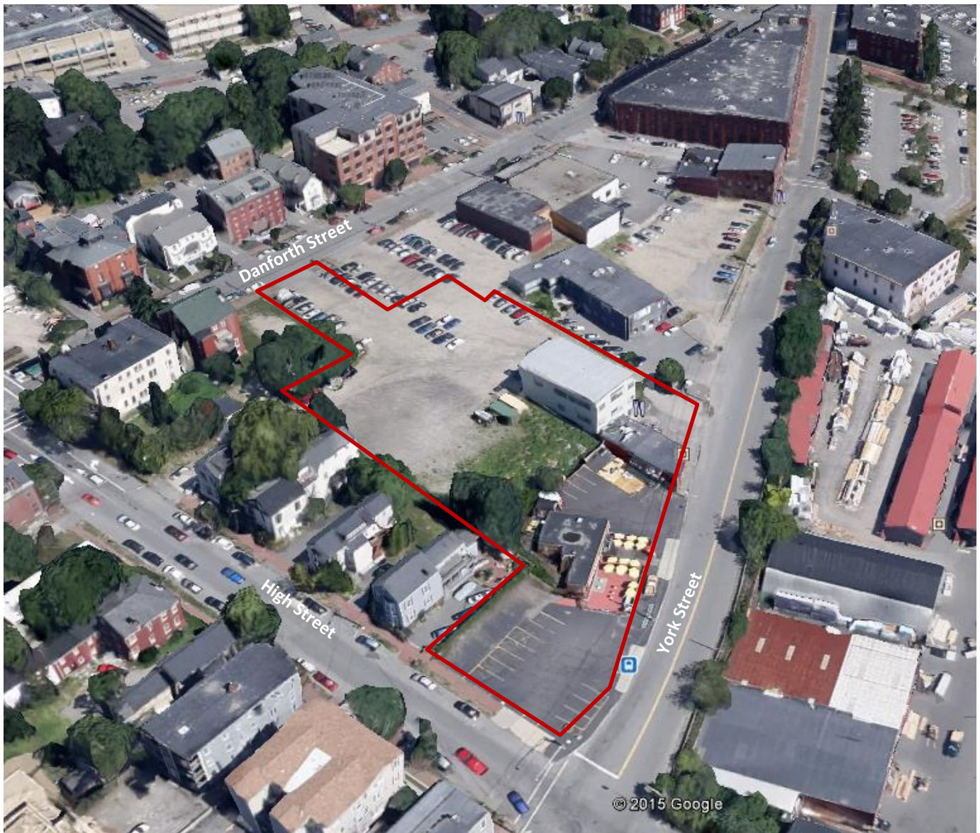
Figure 1: 85-101 York Street site
