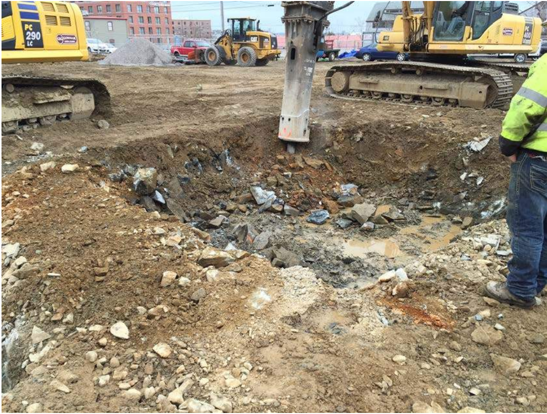
Excavation of Footing D/1
