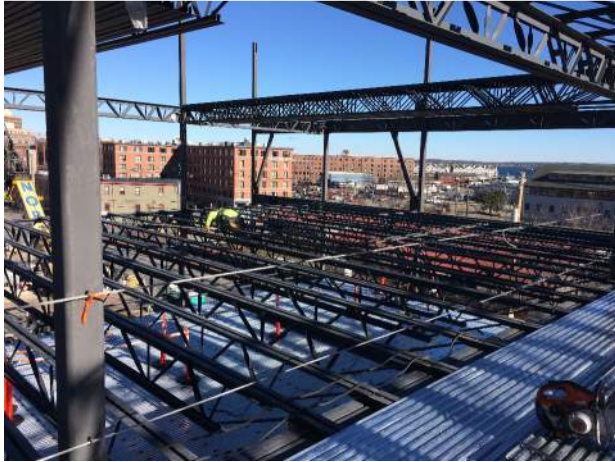
Joists and joist girders.
