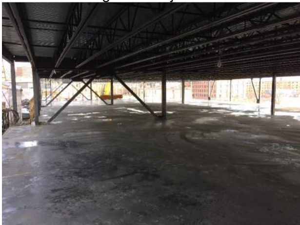
Recently cast concrete slab on decking.
