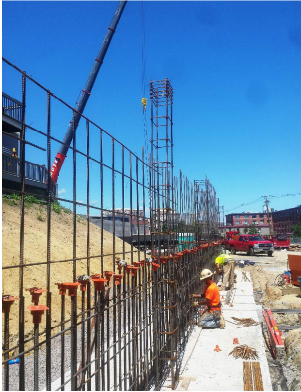
Photo 3) Wall & Pier Reinforcement 15/A to 12/A
