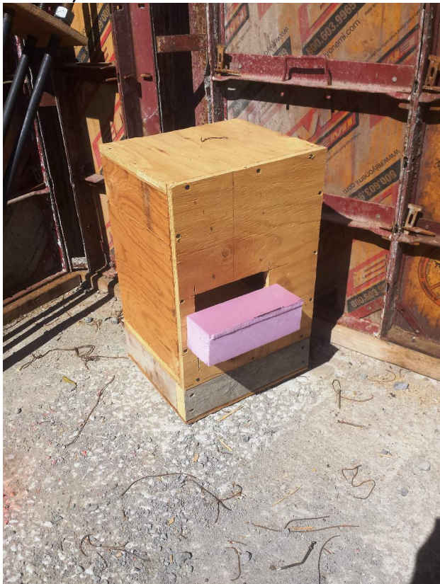
Photos 5 & 6 ) Dropped Pier & Shear Key Boundout, w/ Type AB-2 Anchor Bolts @ A/17
