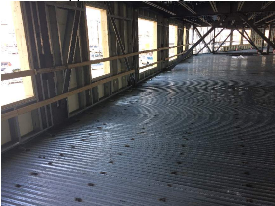
Typical floor deck & welds to framing
