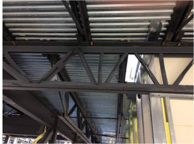
Joists bearing on and welded to girder.
