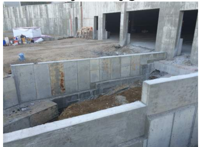
Forms stripped @ mech room area
