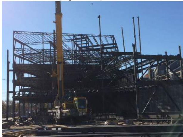
View of progress
