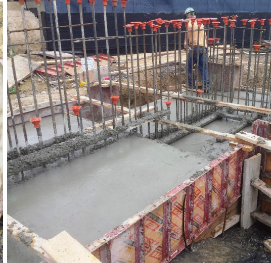
Photo 6) Footing Placement @ 10/A
