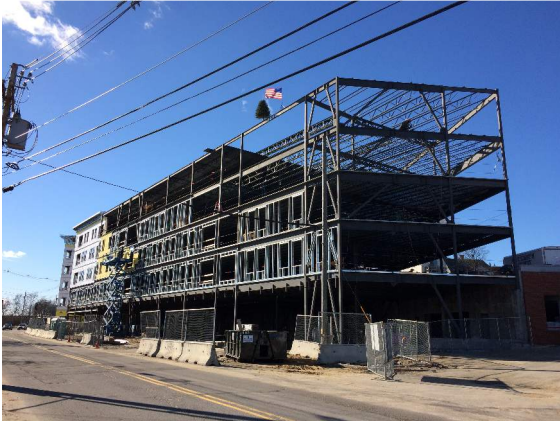
Structural steel progress towards garage
