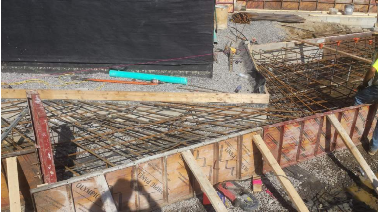
Photo 3) Footing reinforcement near 6.6/B.
