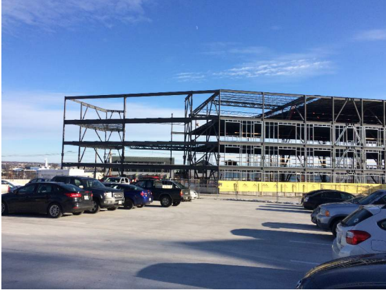
Joist installation progress.
