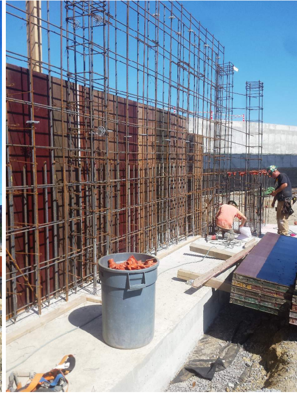
Photo 4) Wall & Pier Reinforcement 11/A to 10/A
