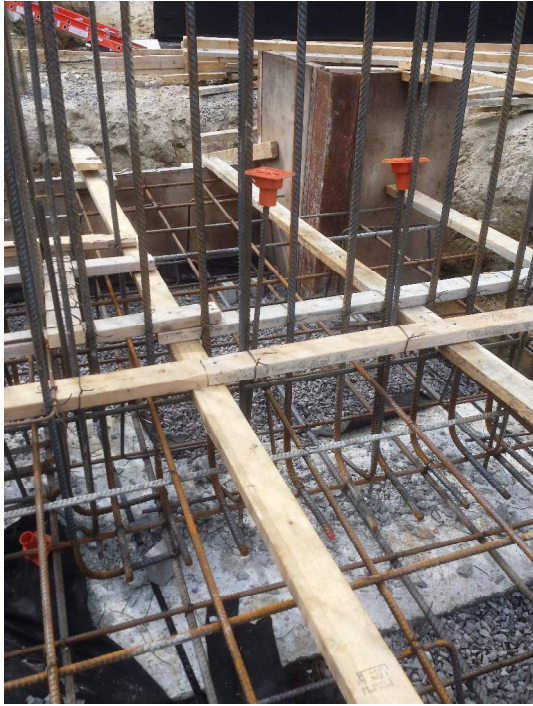
Photo 3) Footing & Wall Reinf. @ 10/A
