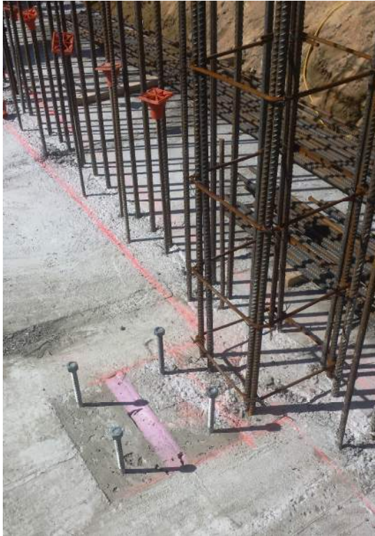
Photo 7) Shear lug bondout (foam), anchor bolts & pier reinforcement @ 6/B.
