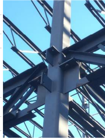
Typical joist girder seat connection.
