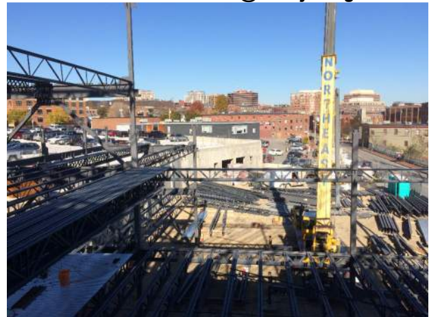
View looking out towards Line 8.
