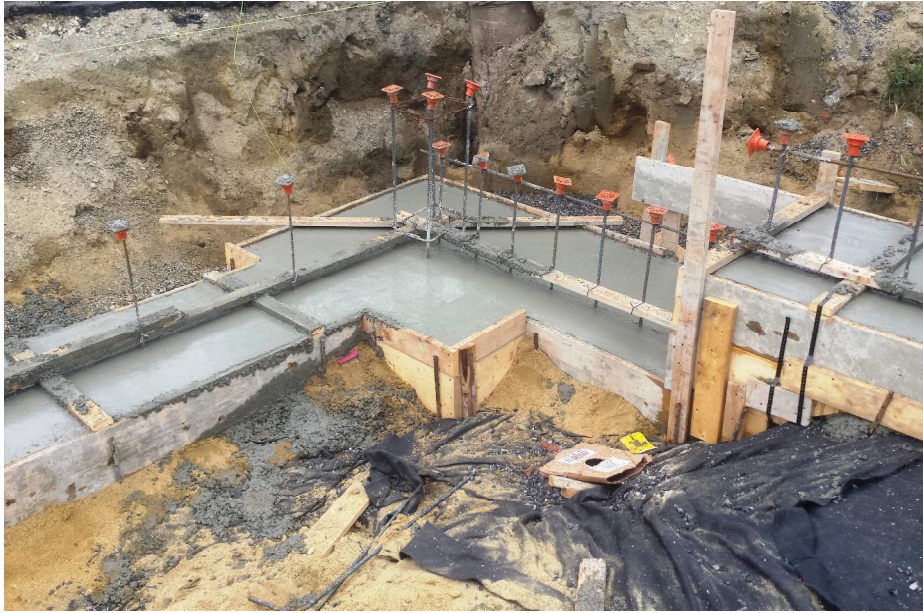
Photo 7) Footing Placement @ 17/G
