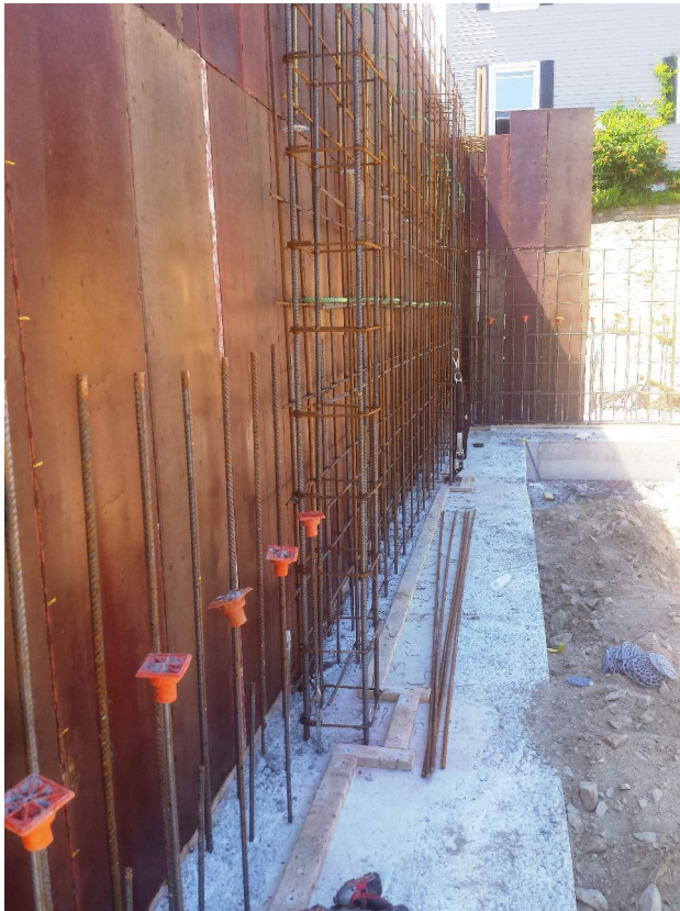
Photo 1) Wall & Pier Reinforcement 17/C to 17/A
