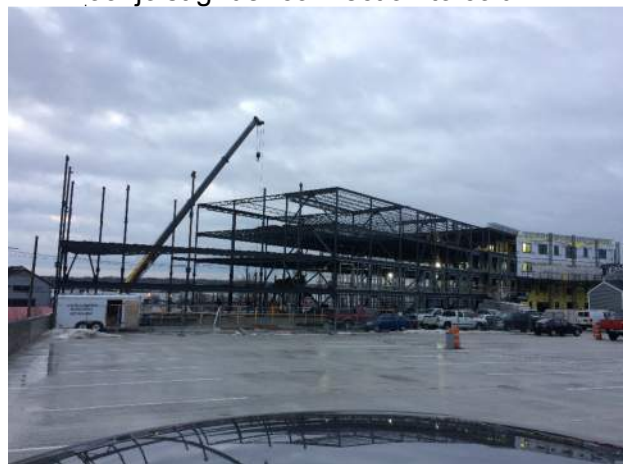
View of progress.
