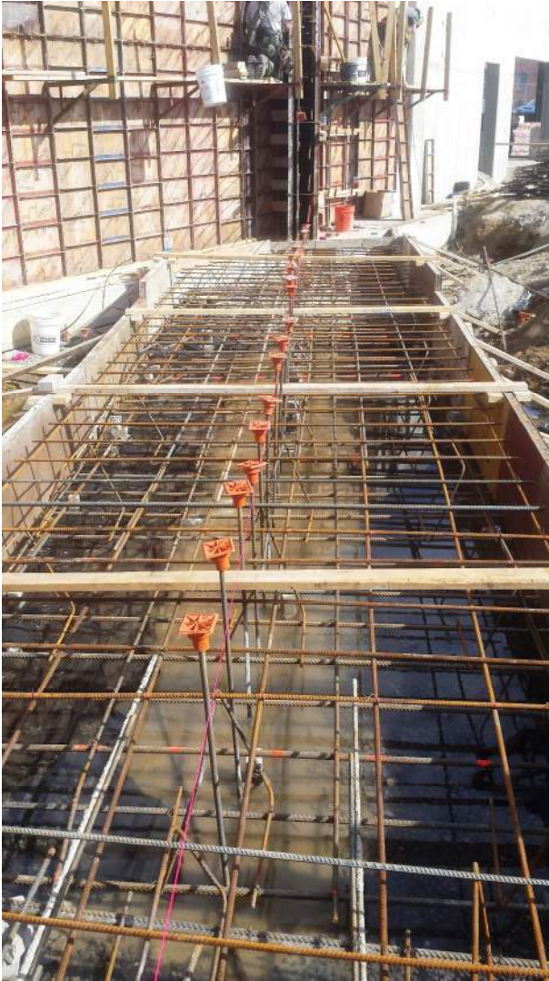
Photo 5) Footing reinforcement from 5/B to 4/B.
