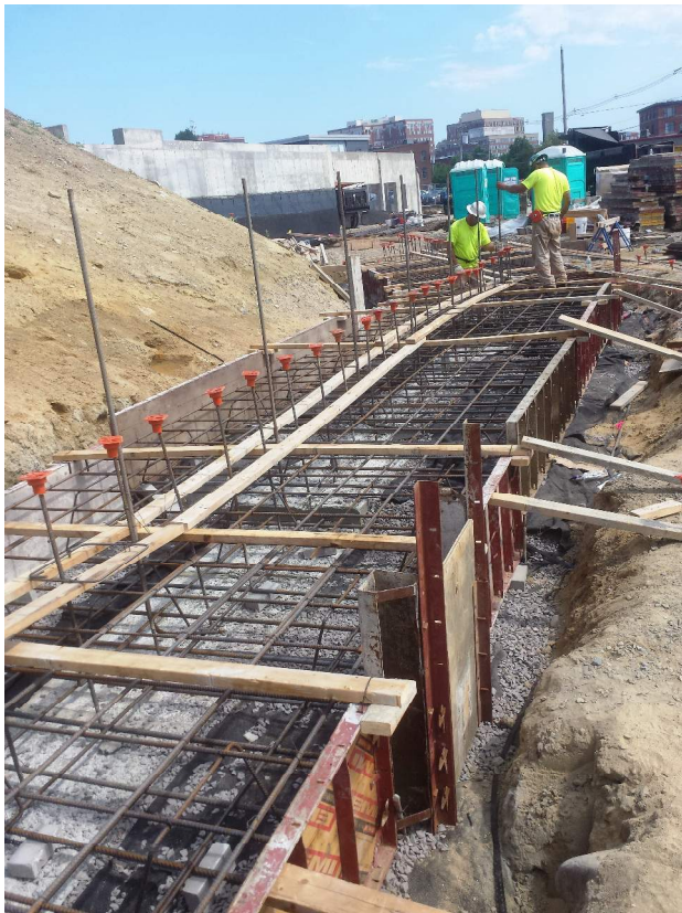
Photo 1) Footing Reinforcement 15/A to 12/A
