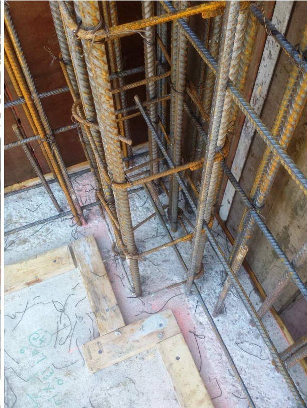
Photo 10) Completed Footing @ 17/A
