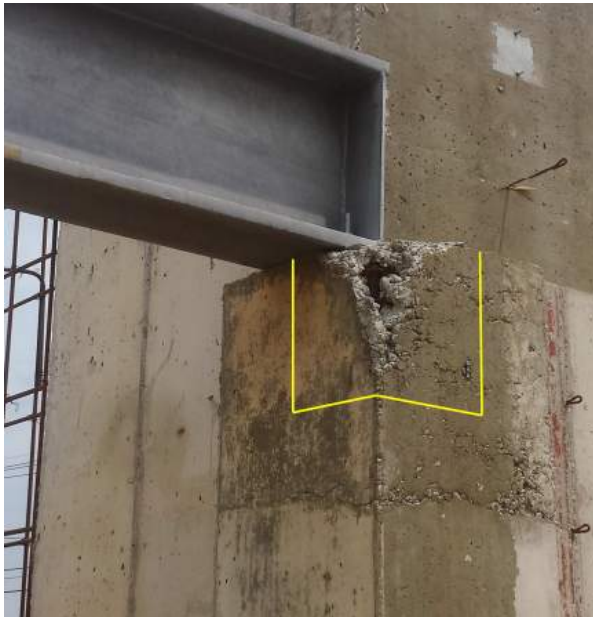
Photo 1) Pier @ H/2 (Garage)
