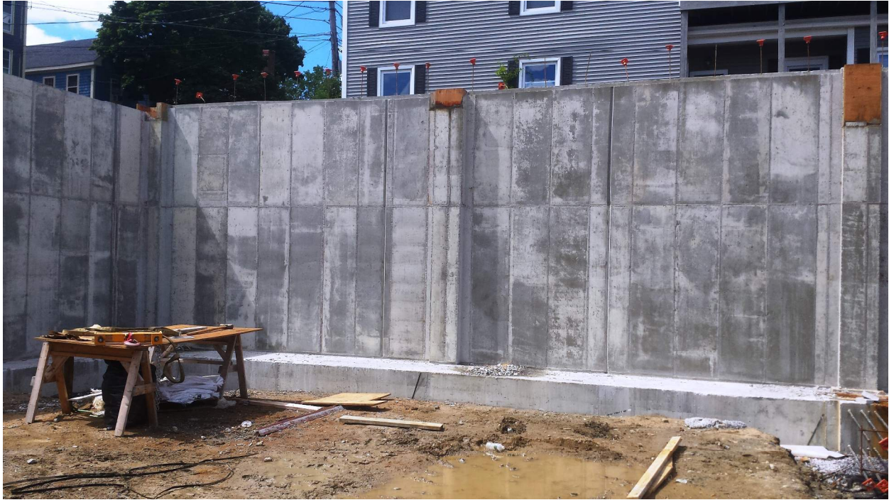
Photo 11) Completed Wall A/17 to A/15
