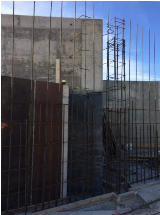
Photo 9) Rebar @ pier & fdn wall intersection
