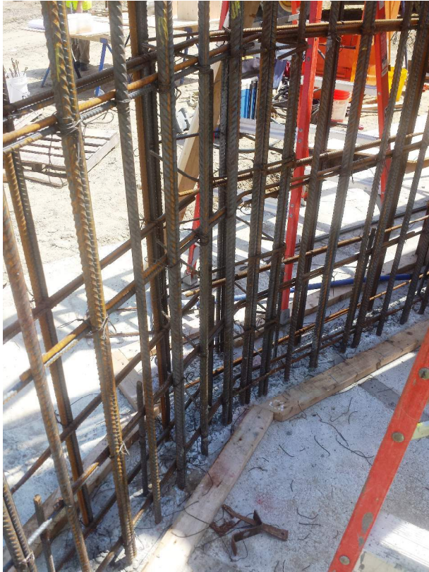
Photo 9) Completed Footing @ 13/A
