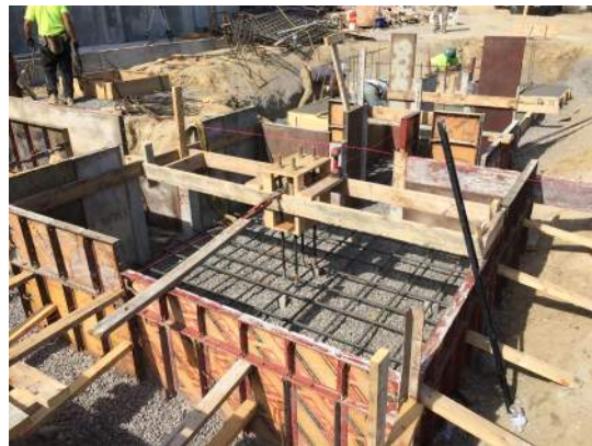
Photo 10) Footing & anchor bolts @ B.9 & C/15-15.4
