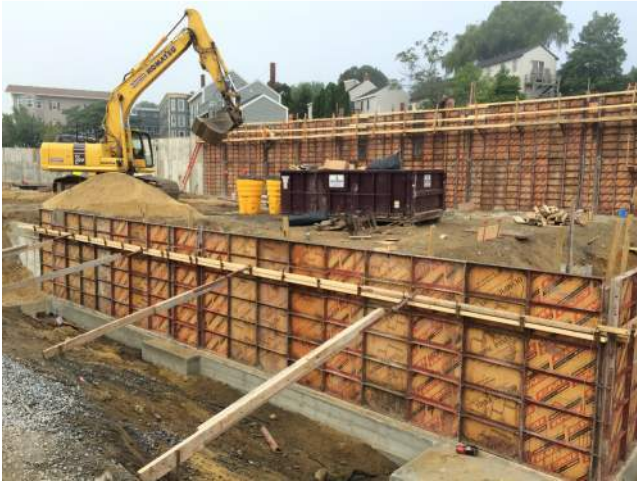
Retaining wall beyond, frostwall front
