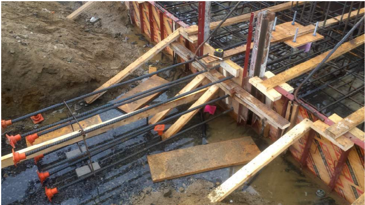
Photo 4) Tie-beam reinforcement, shear lug bondout & anchor bolts @ 8/B.
