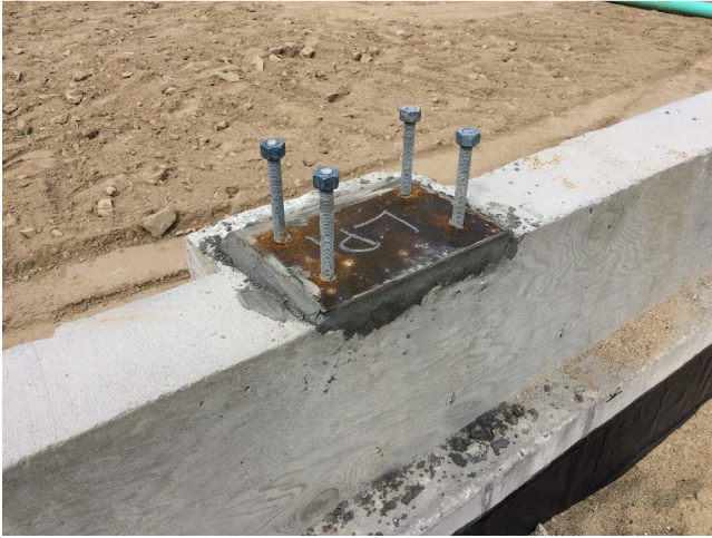
Typical grouted column leveling plate
