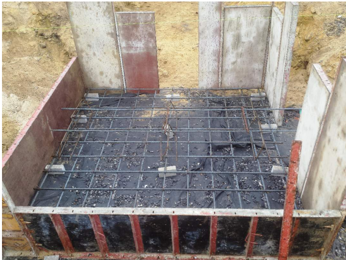
Photo 5) Footing Reinf. @ 15/G
