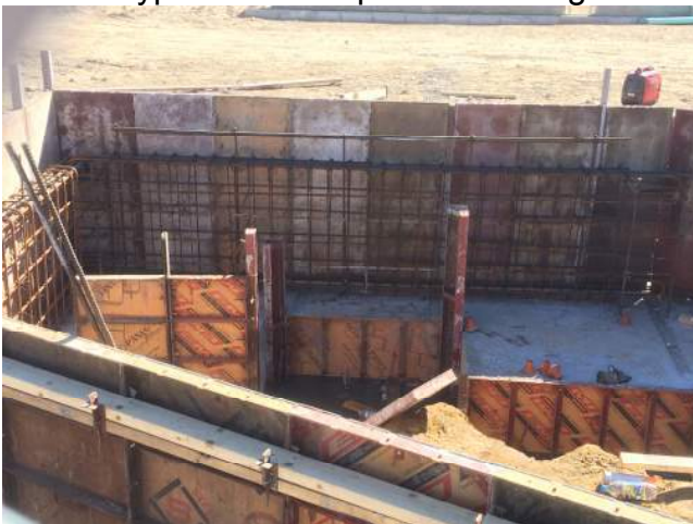
Wall reinforcing @ line 2 (mech rm)
