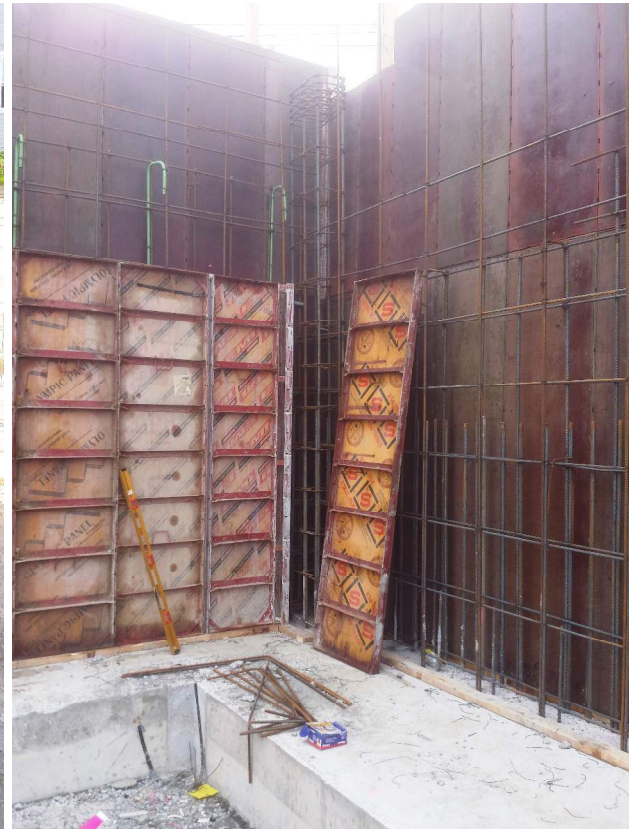
Photo 2) Wall & Pier Reinforcement @ 17/A
