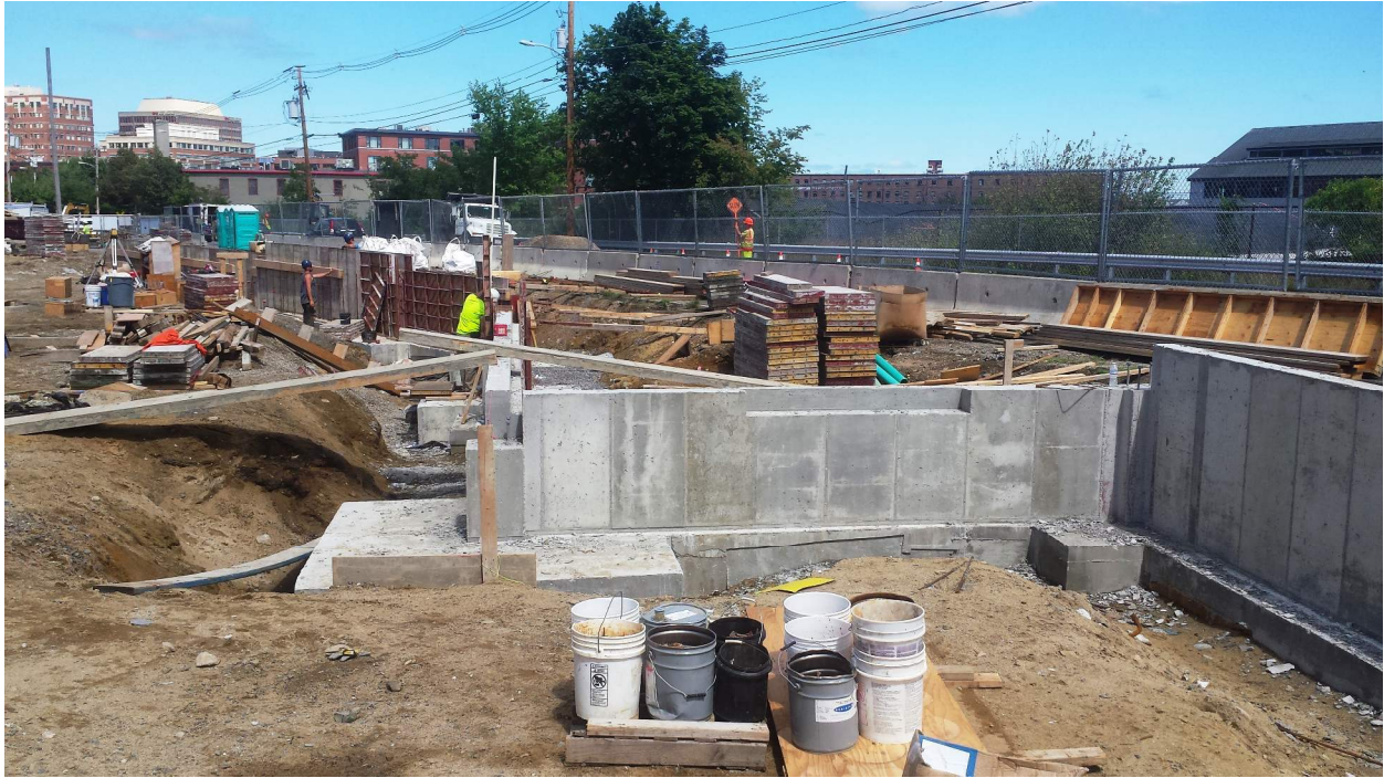
Photo 9) Completed Wall E/13 to G/15
