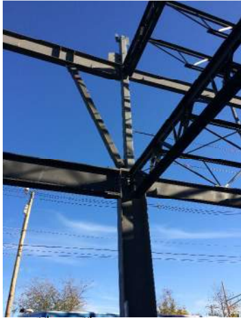
Typical 2 nd & 3 rd floor joists and girders.
