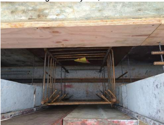
Typical column pier reinforcing
