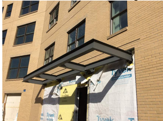
Entry canopy roof frame
