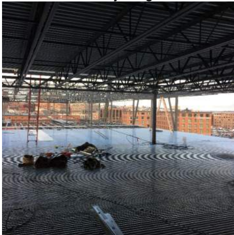
Joist and decking.
