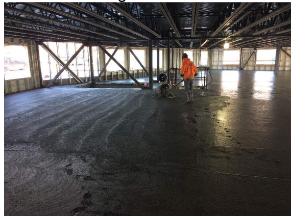
Floor slab finishing
