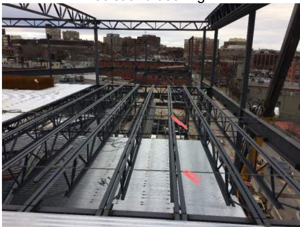
Fifth floor joist and roof joists above prior to placement.
