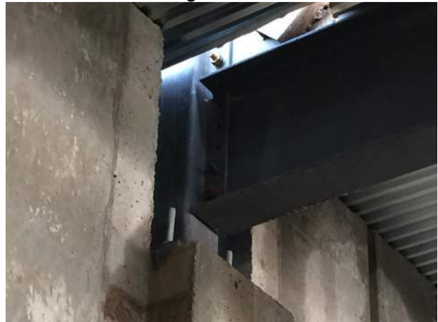
Second floor beam connection to column bearing on concrete pilaster.
