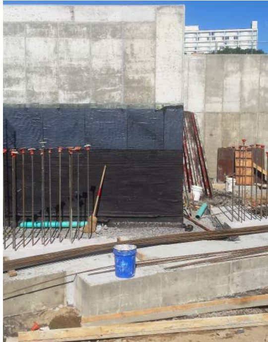
Photo 8) Completed footing near 6.6/B
