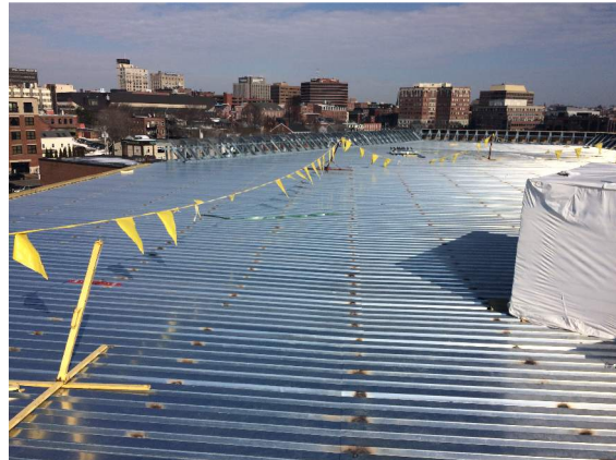
Roof deck & welds to framing
