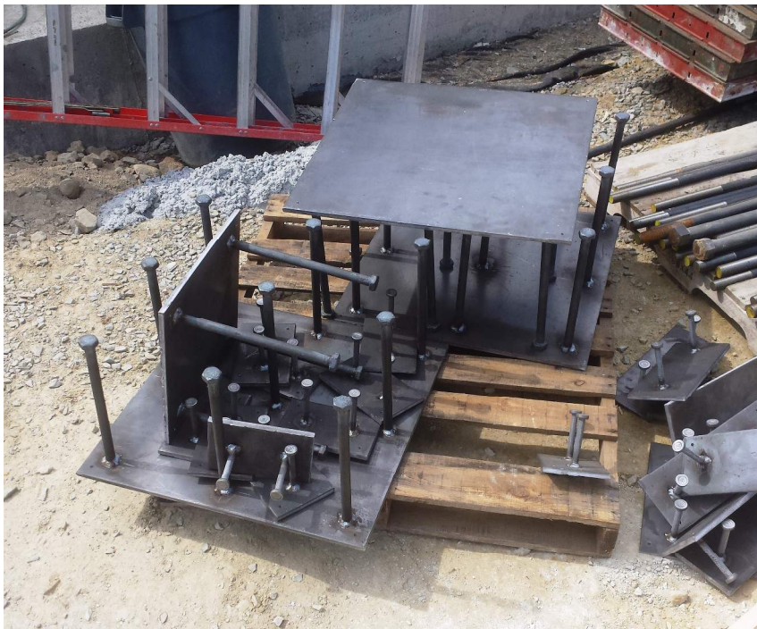
Photo 8) Embed Plates w/ Headed Studs
