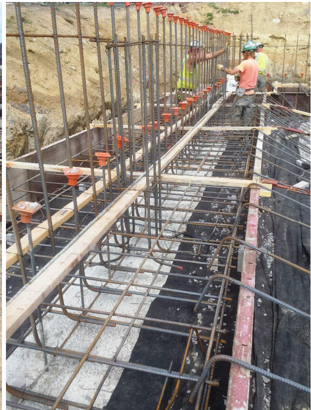
Photo 2) Footing, Pier & Wall Reinf. 17/C to 17/A
