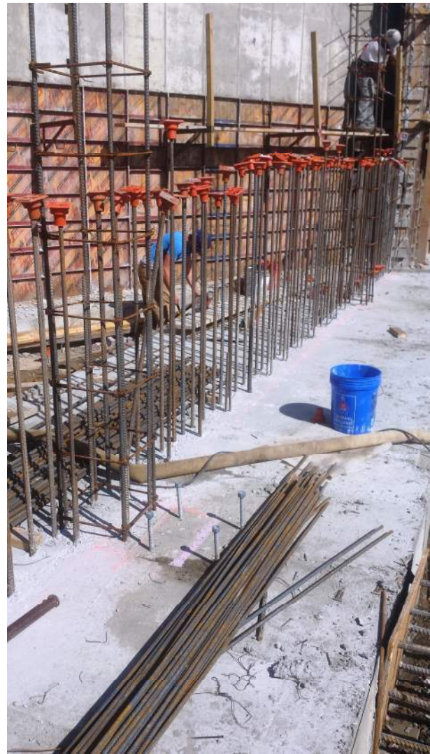
Photo 6) Completed footing from 6/B to 4/B.
