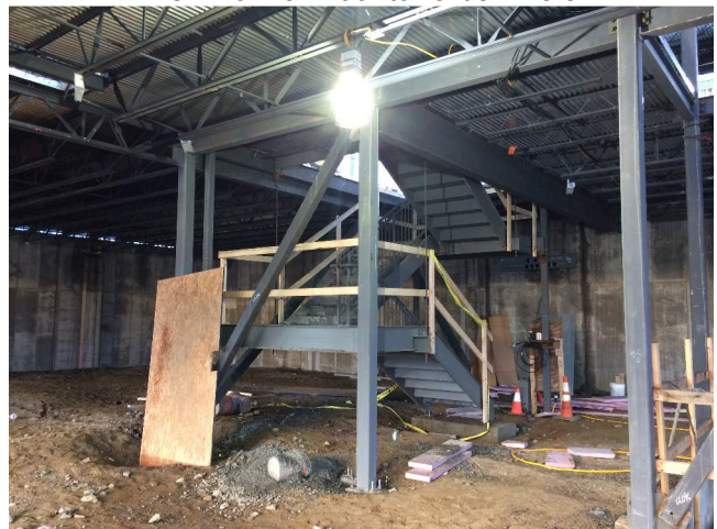
View at basement stair
