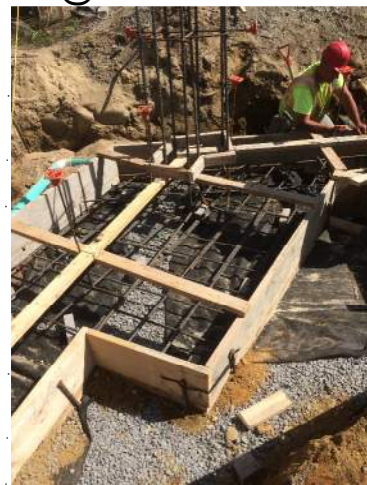
Column footing reinforcing @ lines F/Y3/1
