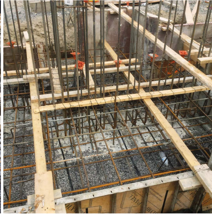
Photo 4) Footing & Wall Reinf. @ 10/A
