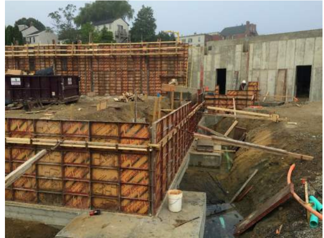
Frostwall @ intersection of lines F & 4
