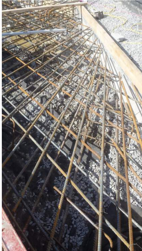
Photo 2) Footing reinforcement, w/ longitudinals drilled & epoxied into garage footing near 6.6/B.
