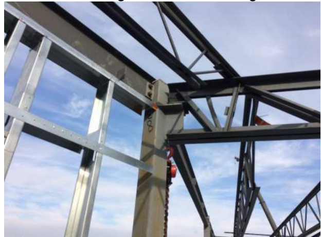
Roof joist girder connection to column.
