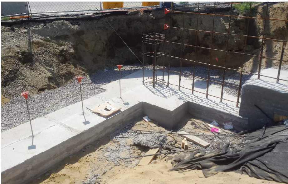
Photo 8) Completed Footing @ 17/G
