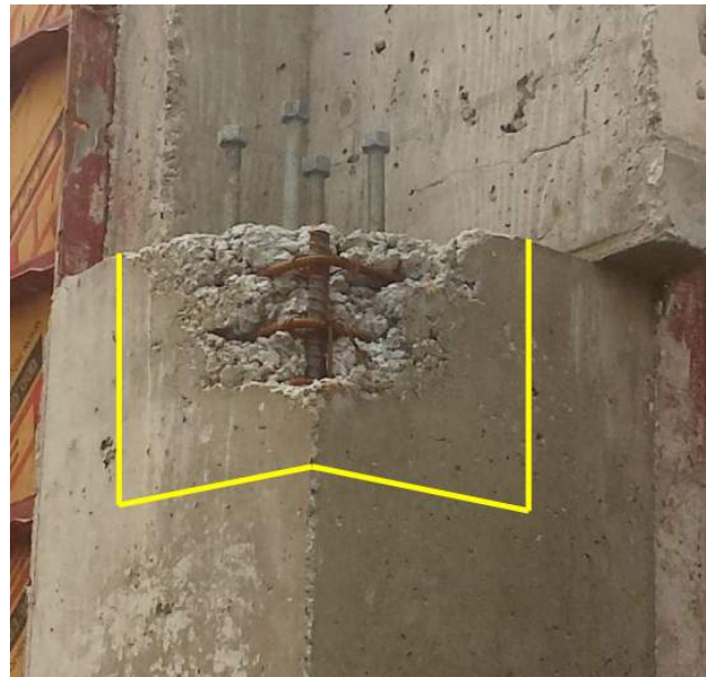
Photo 2) Pier @ Y1/X4 (Building)
