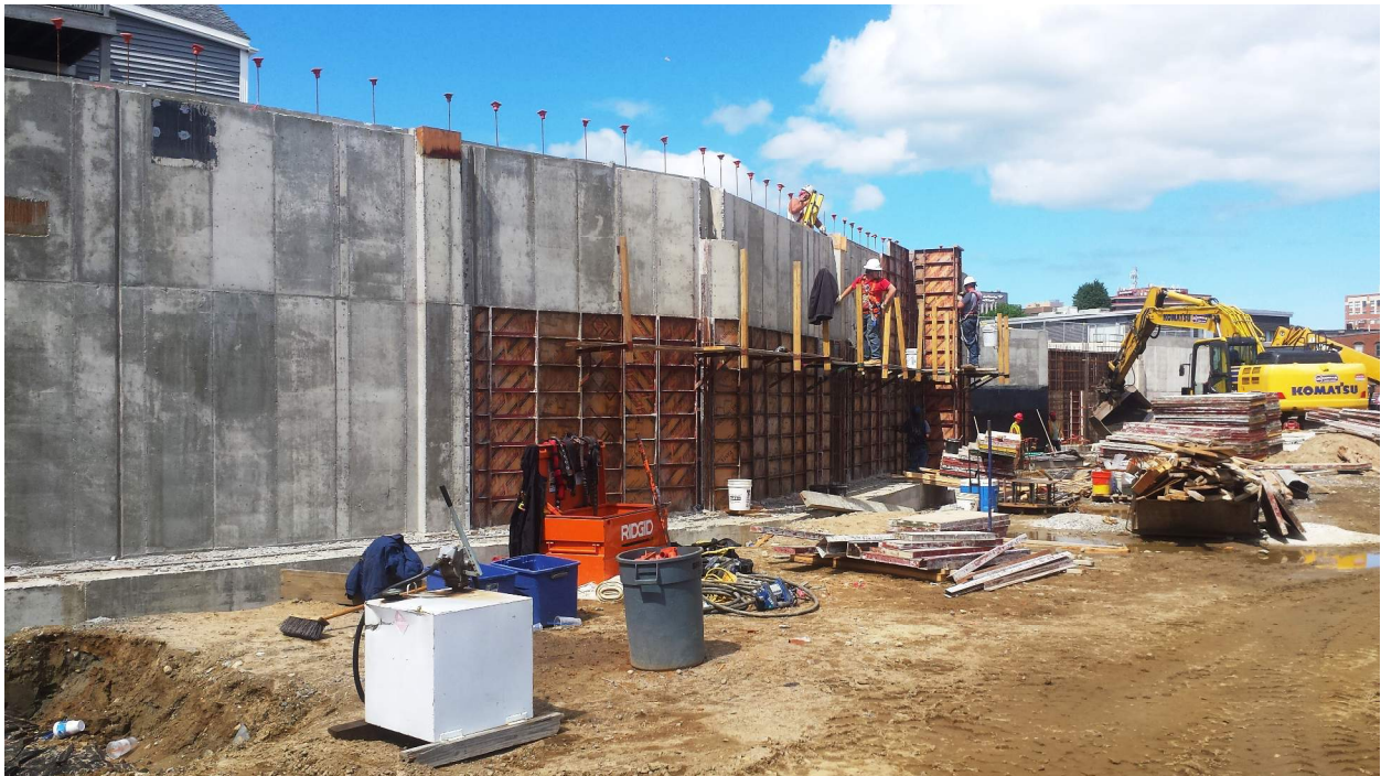
Photo 12) Completed Wall A/14 to A/11
