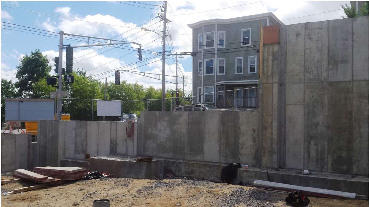
Photo 10) Completed Wall G/17 to D.2/17
