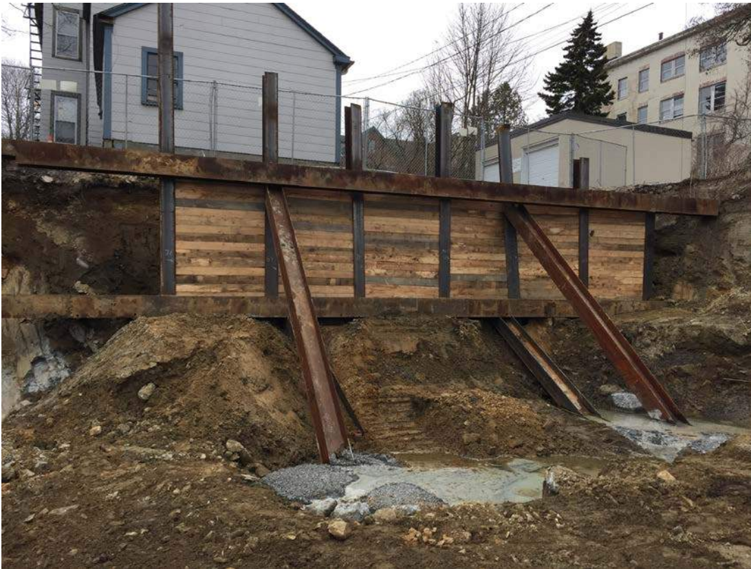
Soldier Pile Wall Installed by HBF1
