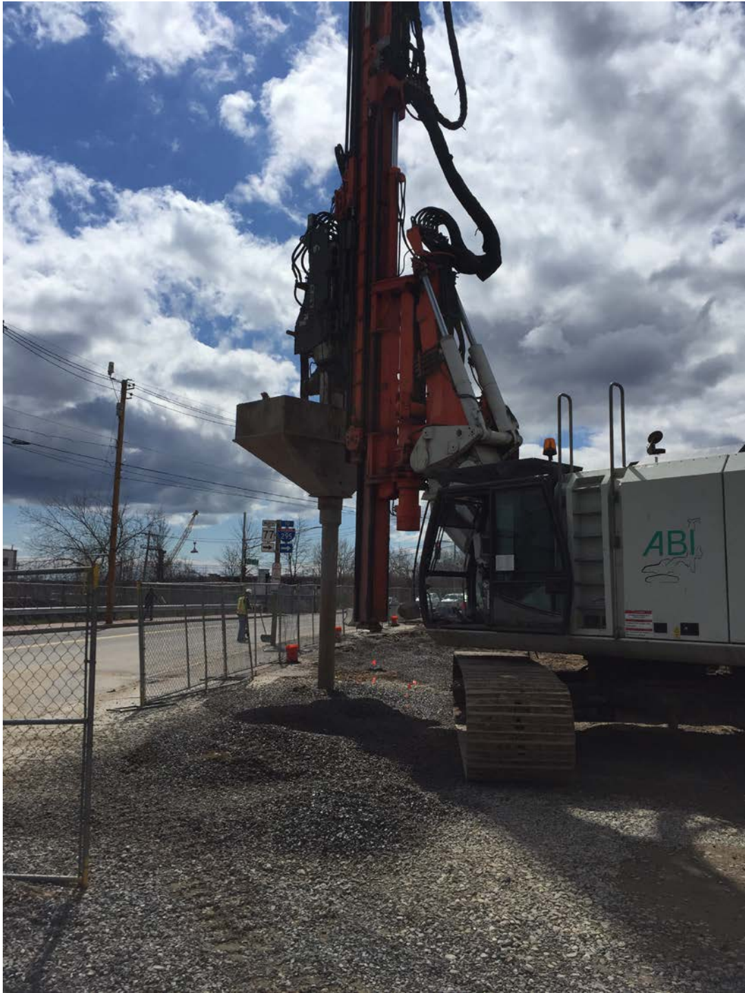
Installing RAPs
