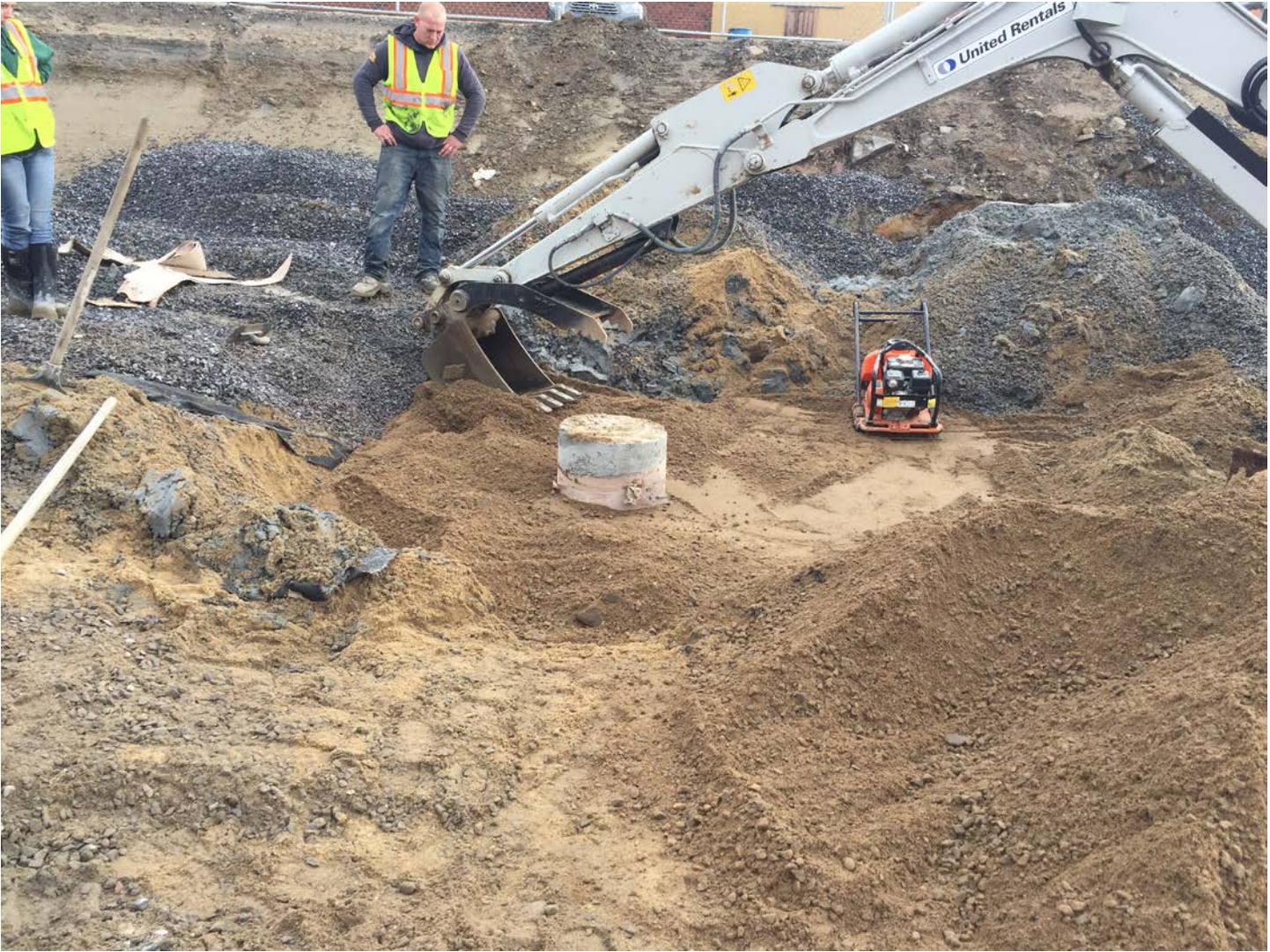
Preparing Test RAP #2
