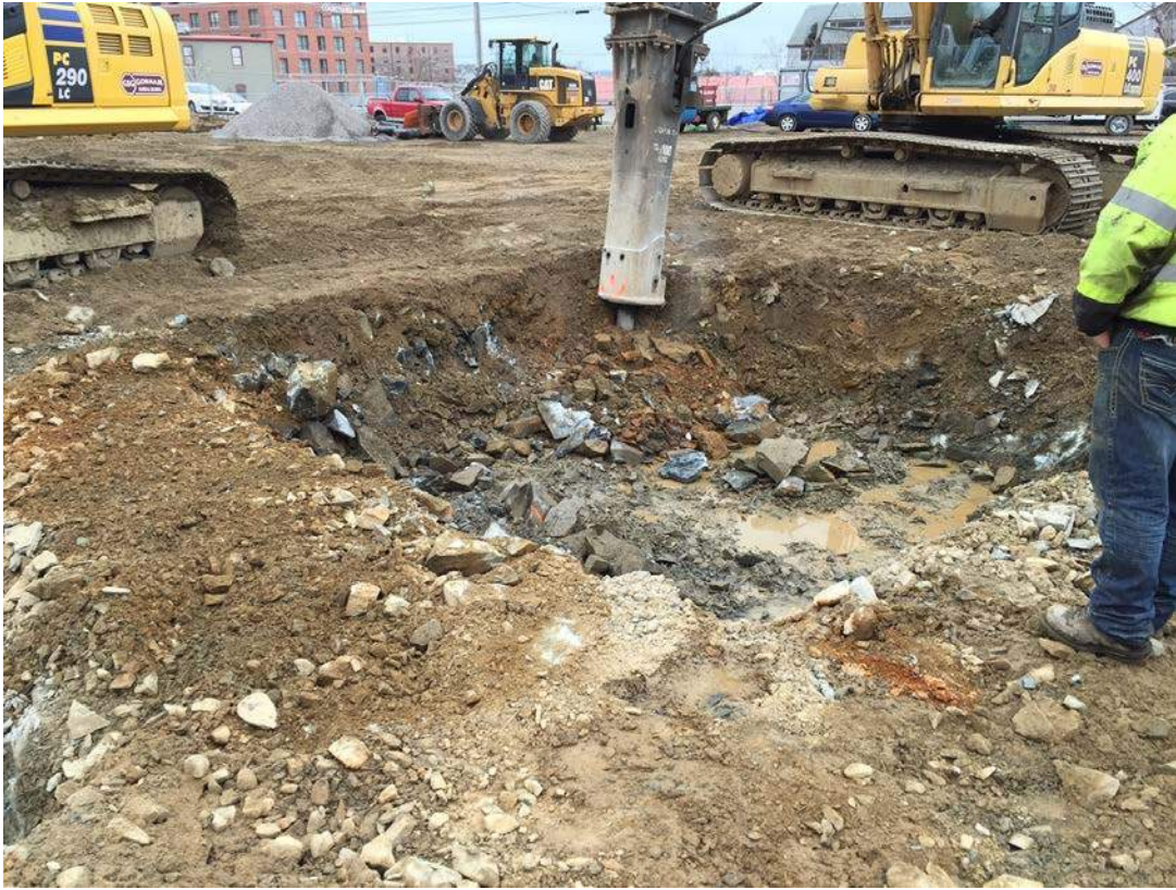
Excavation of Footing D/1
