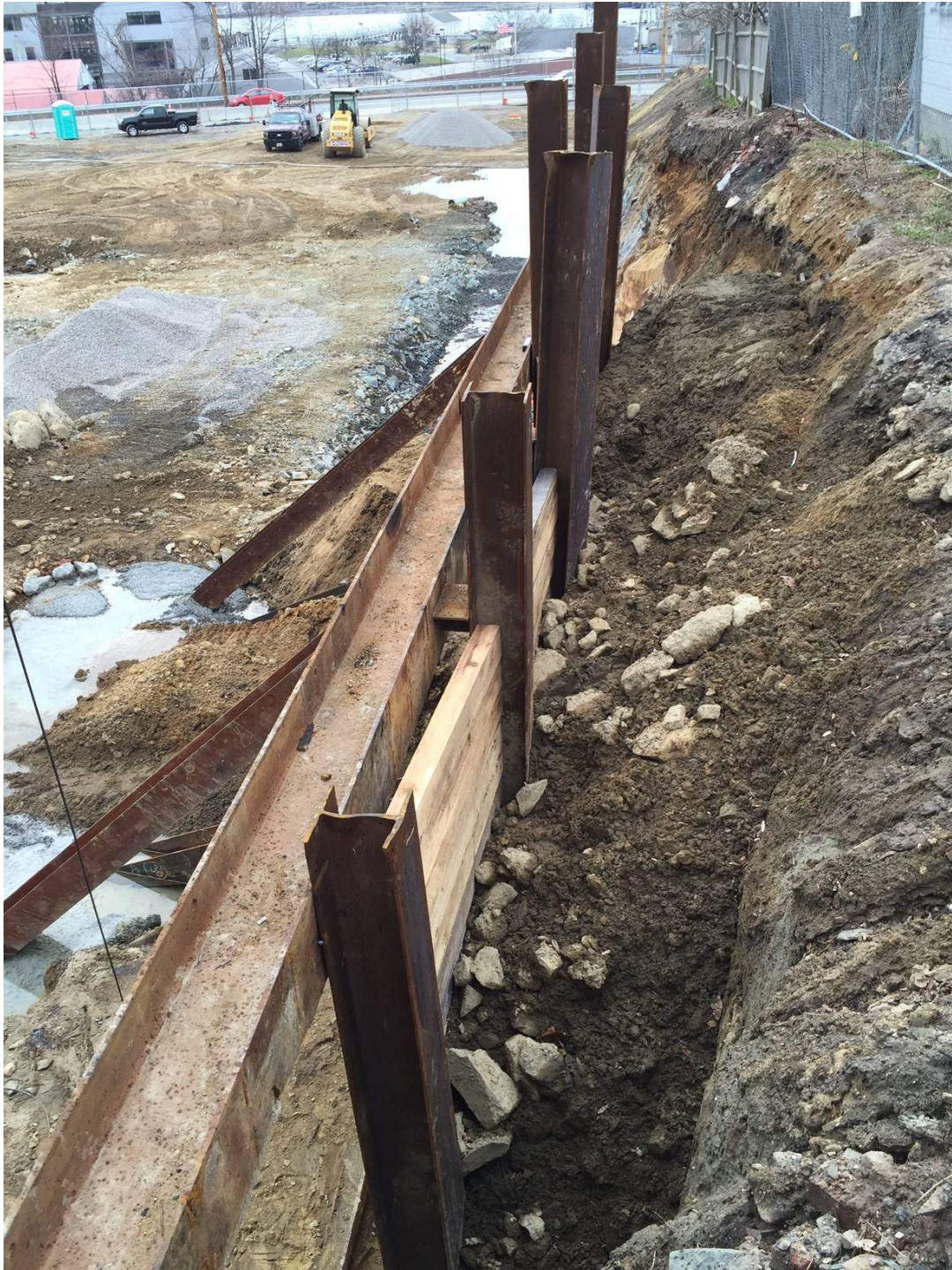
Backfill of Soldier Pile Wall
