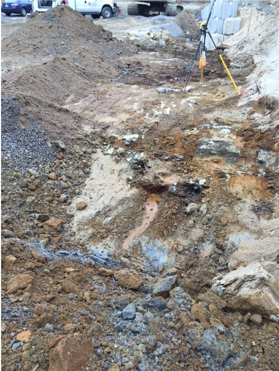
Excavation Along Northern Perimeter Foundation Between RAPs 341 and 346
