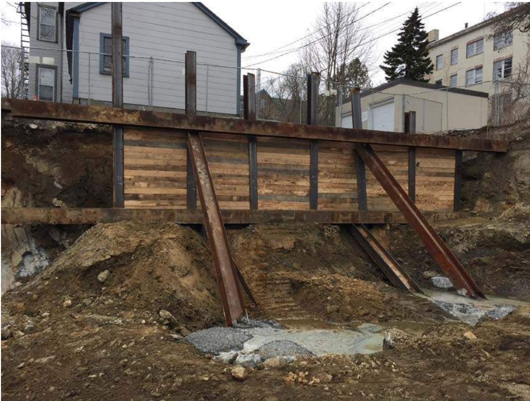
Soldier Pile Wall Installed by HBF1
