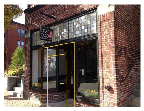
The dimensions of this opening are 68" wide by 96" tall. Door is 36x80, swings outward Side panels are 16x96 Transom panel is 36x16
