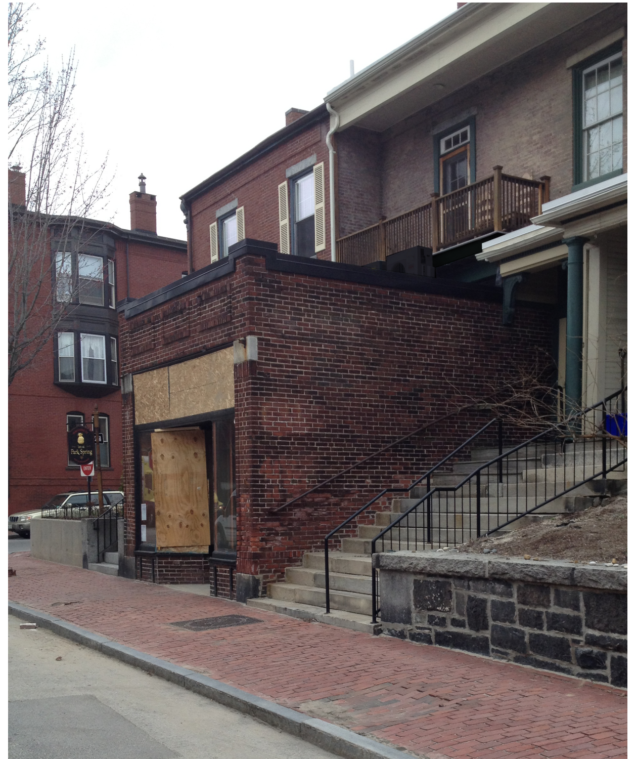
2 Black Painted Heat Pumps
