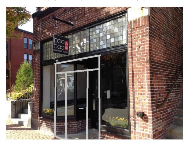
The dimensions of this opening are 68" wide by 96" tall. Door is 36x80, swings outward Side panels are 16x80 Top panel is 68x16
