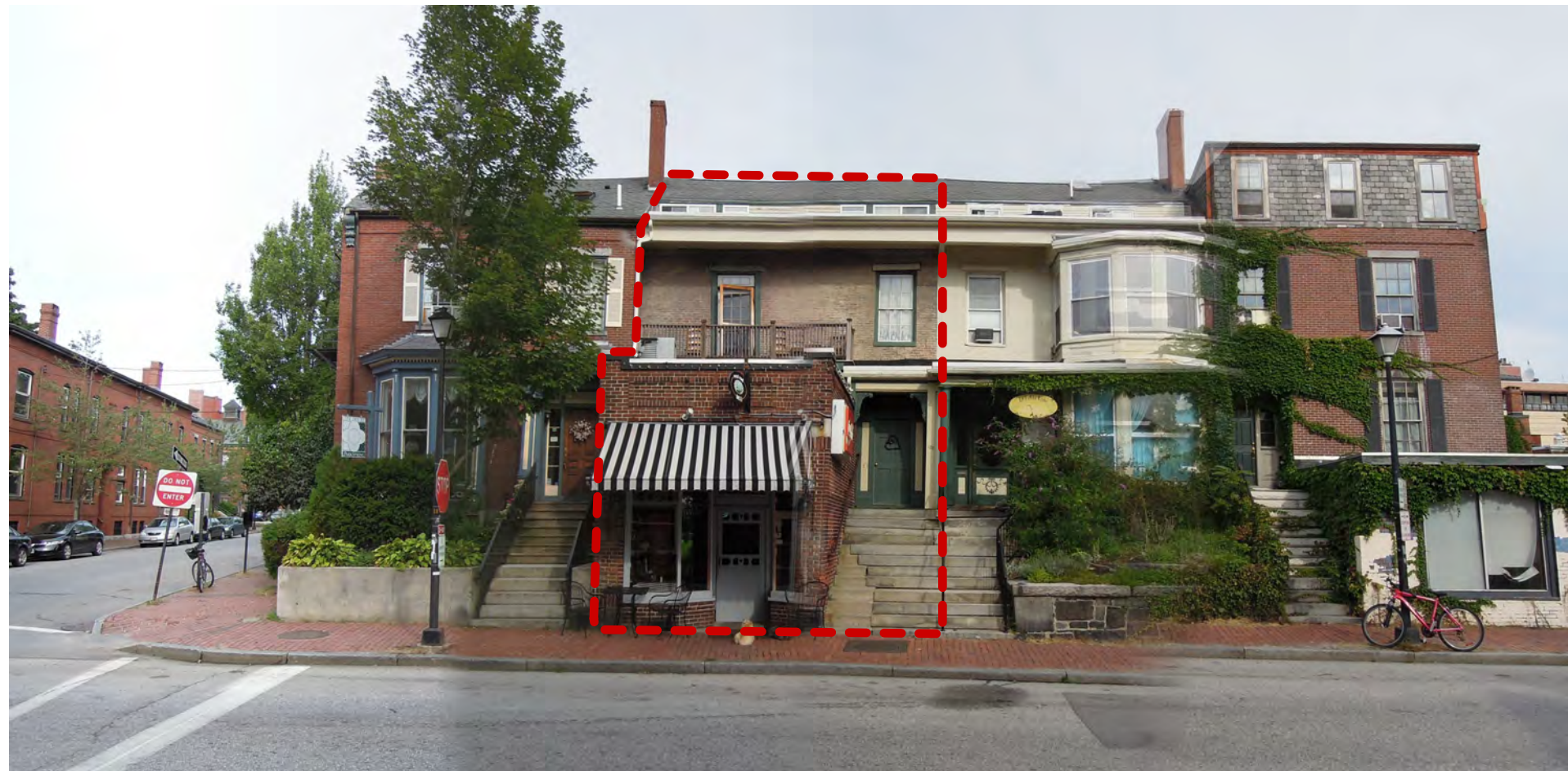
EXISTING SPRING ST FACADE
