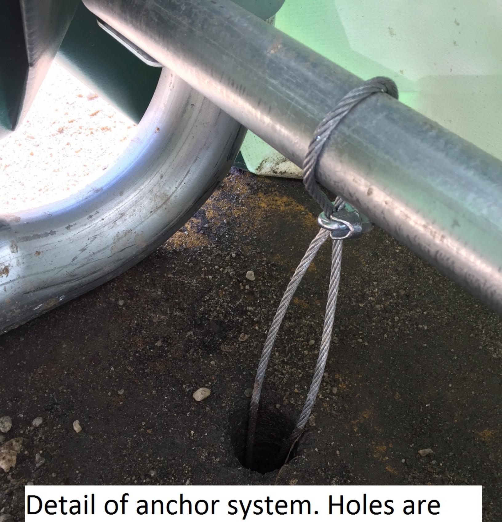
Detail of anchor system. Holes are 18" deep. Wire is attached to base and then attached to heavy duty anchors driven into the holes. 6 anchors per side.
