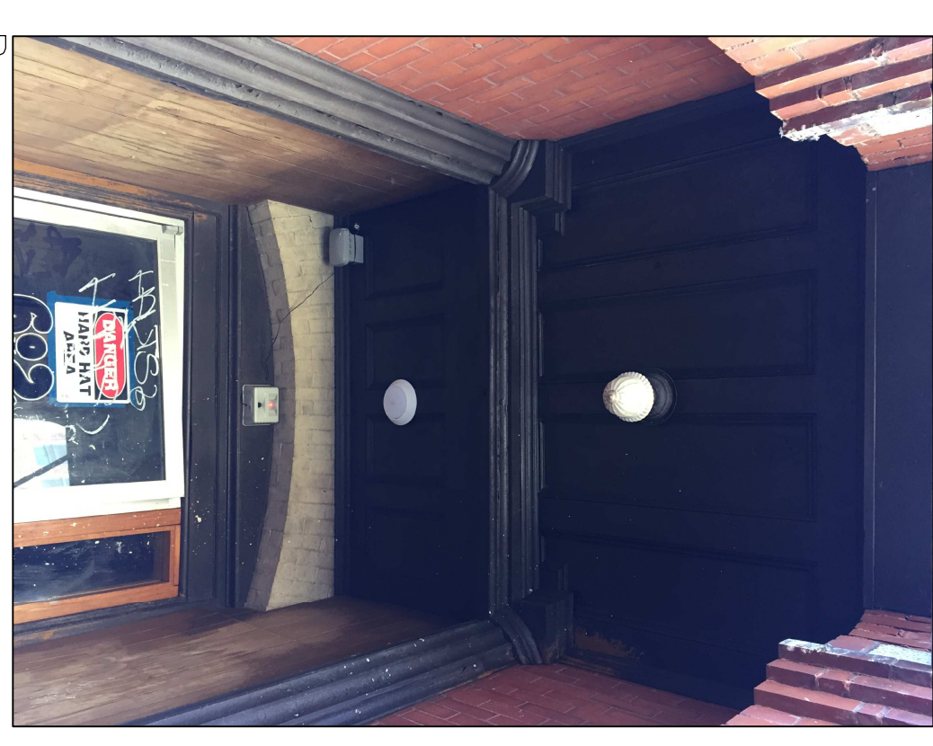
603 ENTRY CEILING Residential Apartments
