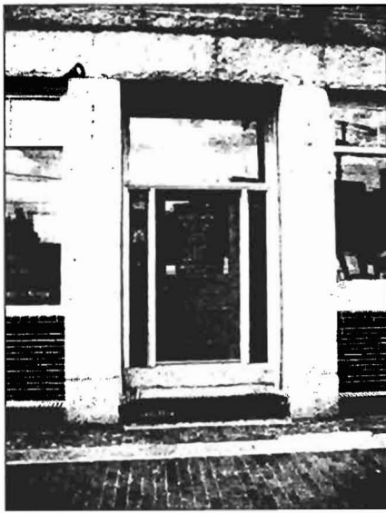
SOUTH ENTRY STAIR
