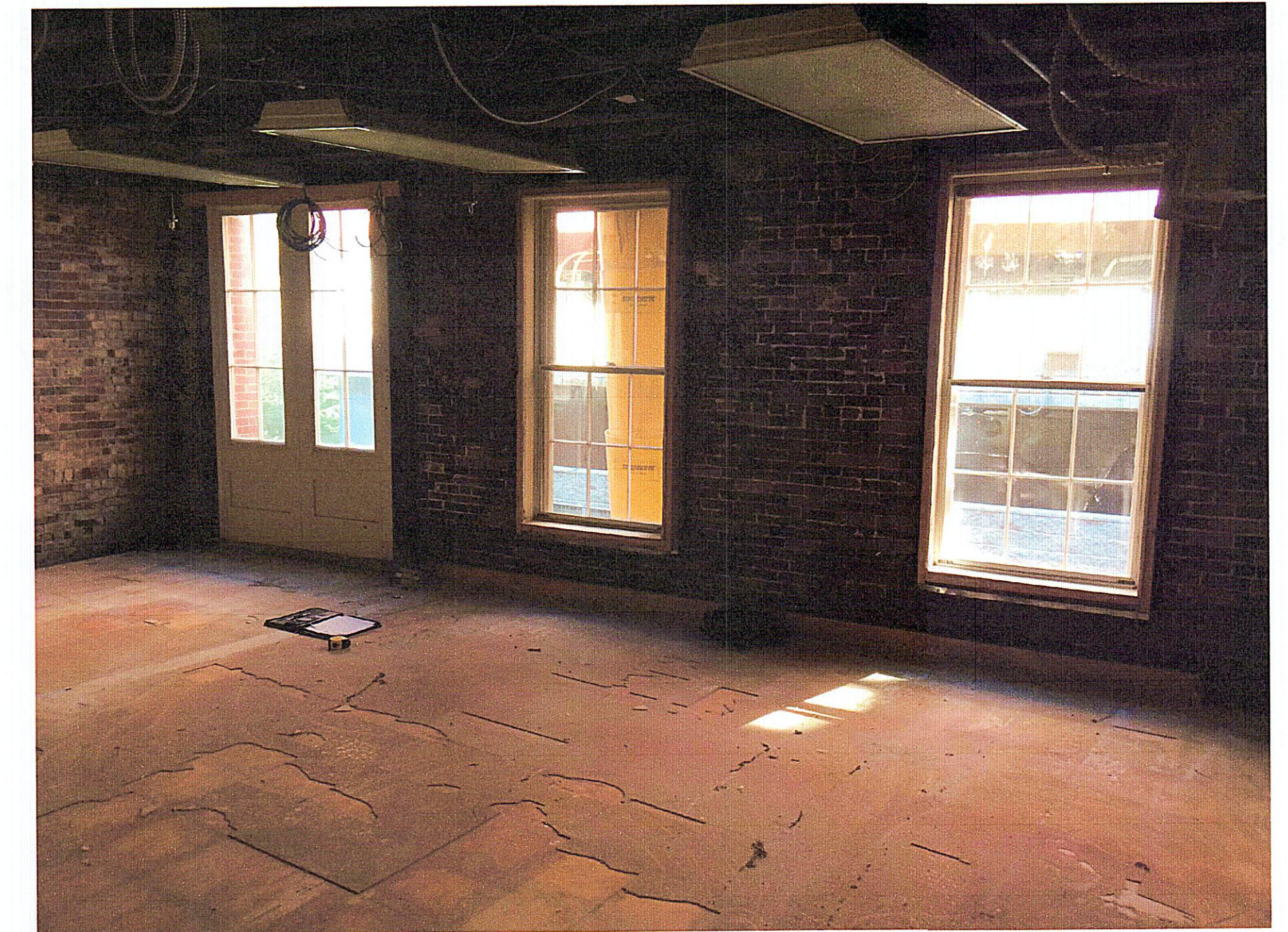
TYPICAL INTERIOR - WEST
