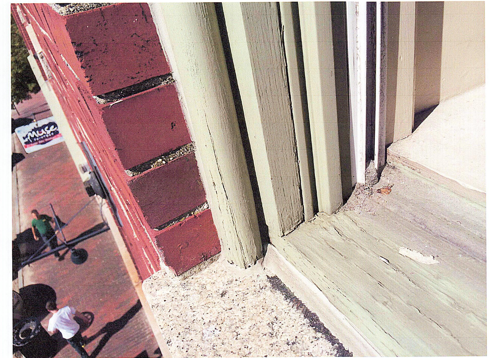
TYPICAL EXISTING WINDOW FRAME
