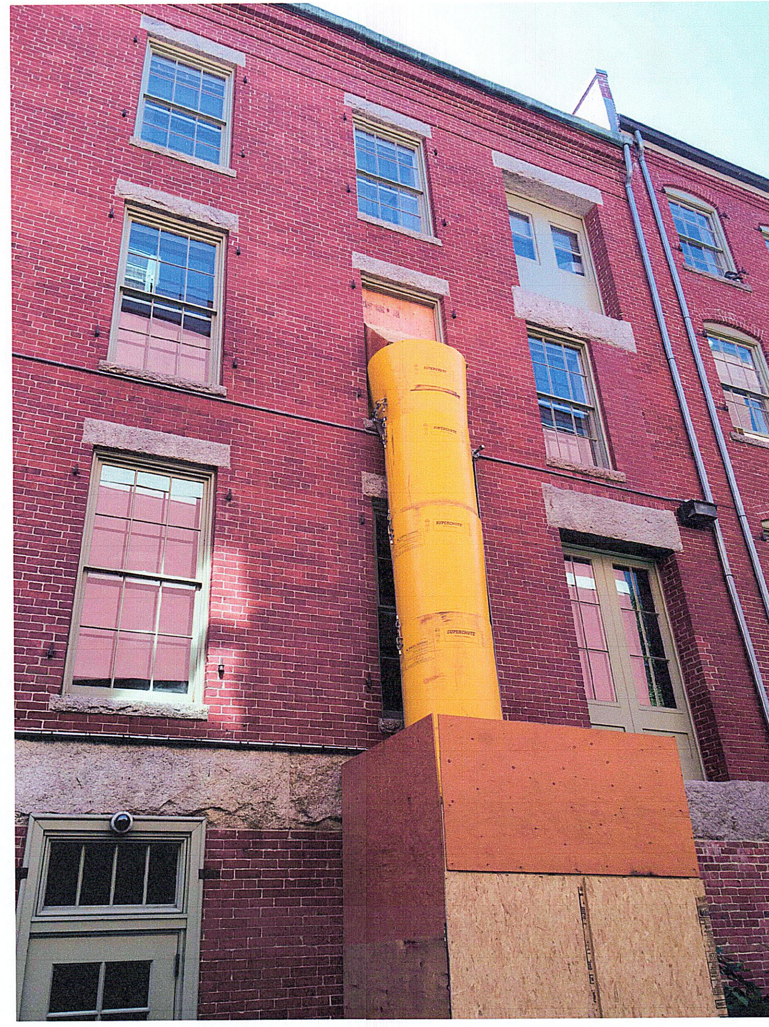
TYPICAL REAR SERVICE DOORS & WINDOWS - WEST
