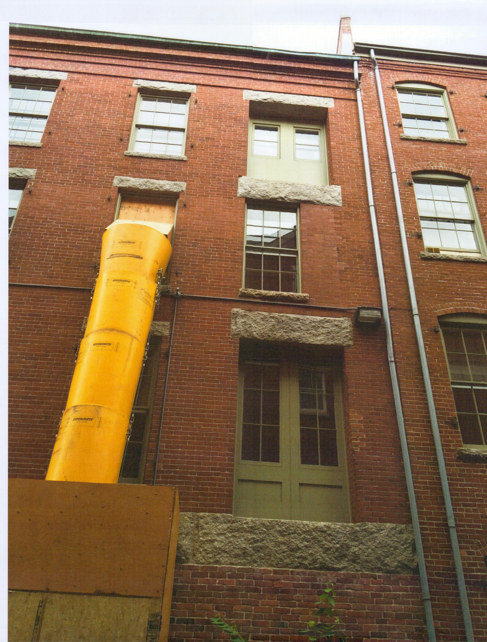
TYPICAL REAR SERVICE DOORS & WINDOWS – WEST
