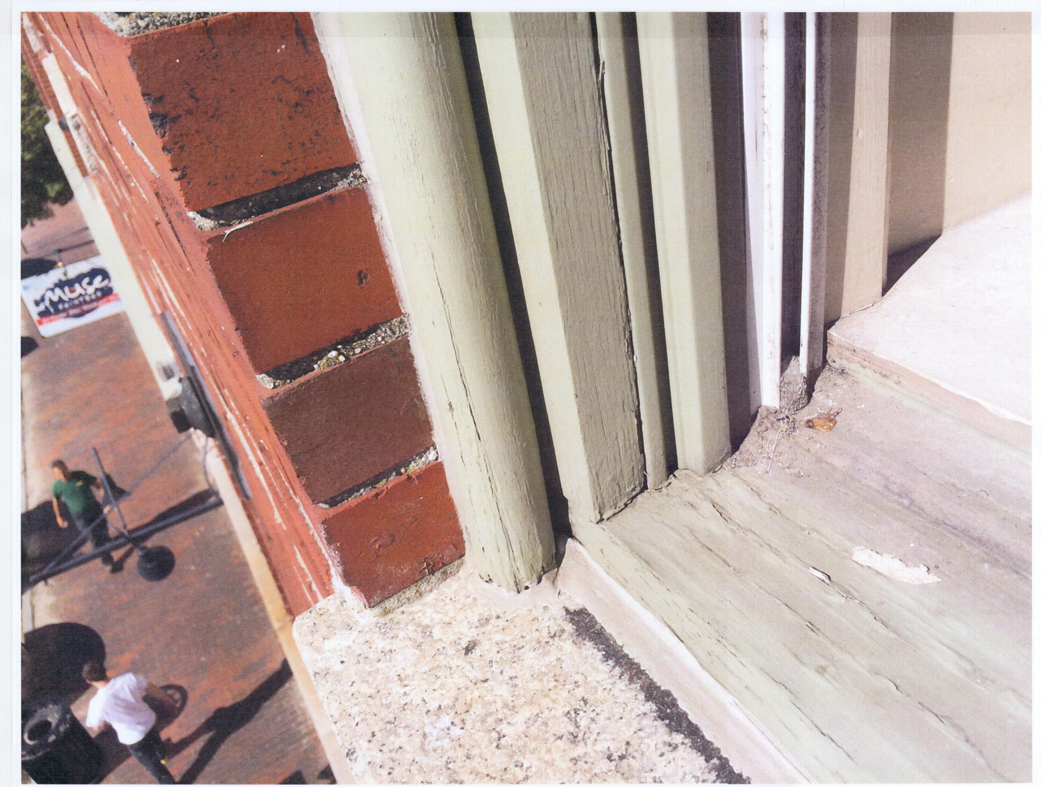
TYPICAL EXISTING WINDOW FRAME
