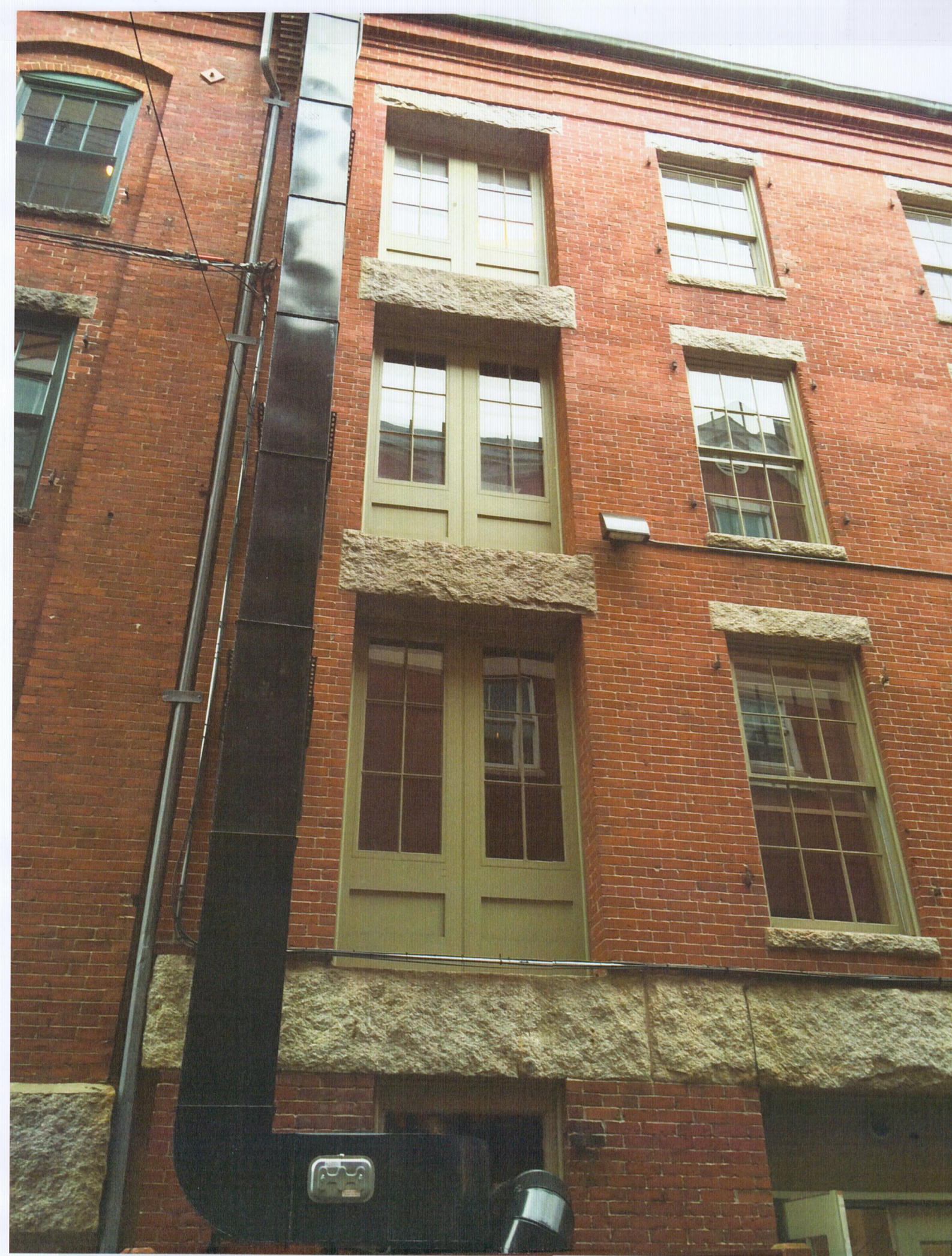
TYPICAL REAR SERVICE DOORS & WINDOWS – EAST
