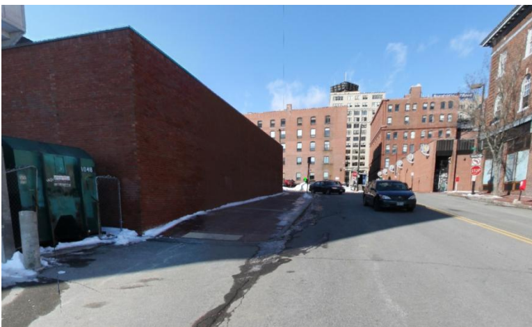
Image 2 View on Center Street toward Congress Street. Proposed building addition will be located in portion of the existing brick wall. Building height will increase by approximately 12'-5".
