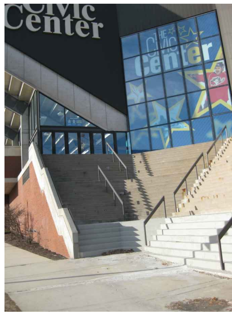
N1 SITE PHOTO
