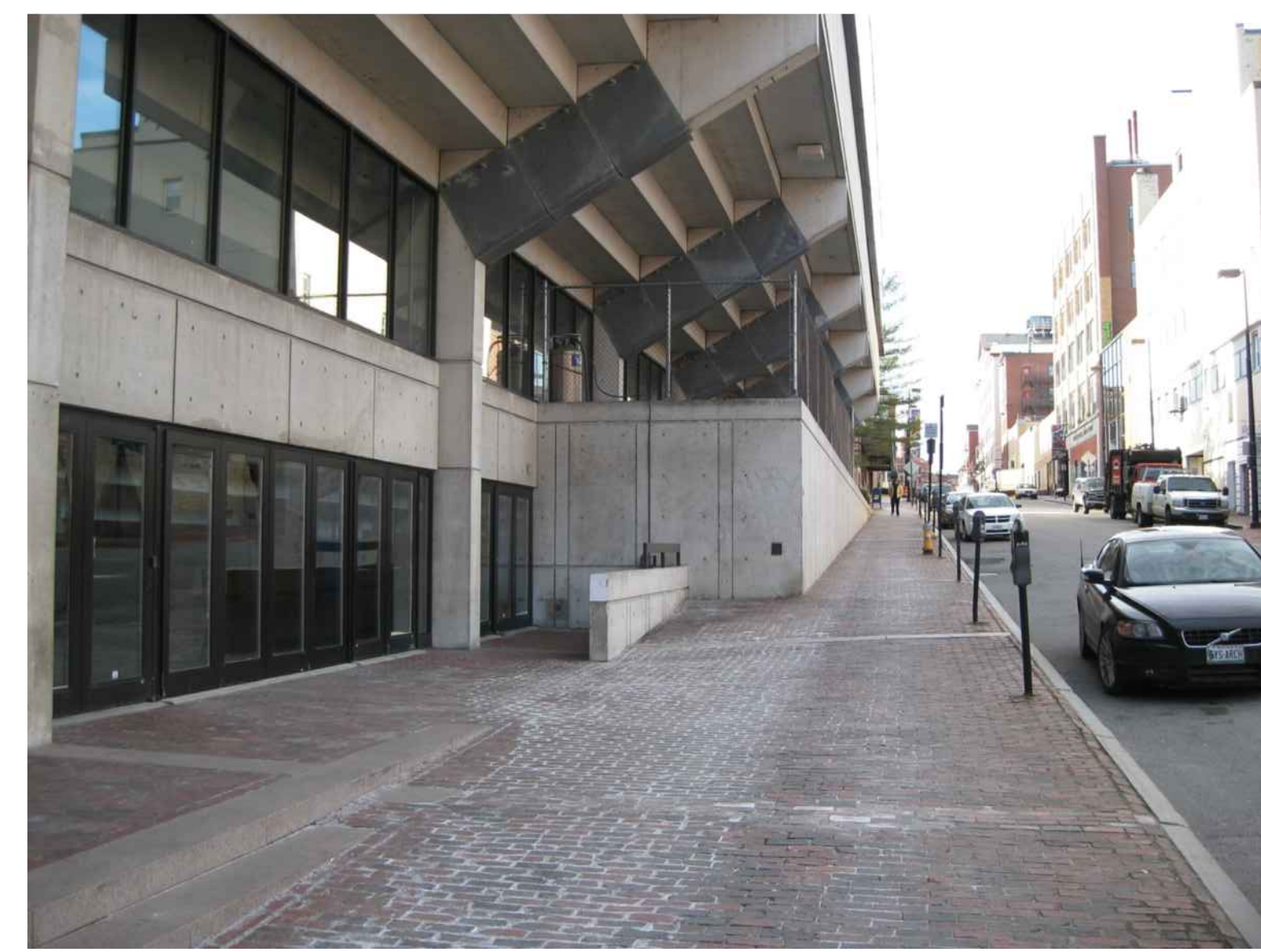
N10 SITE PHOTO
