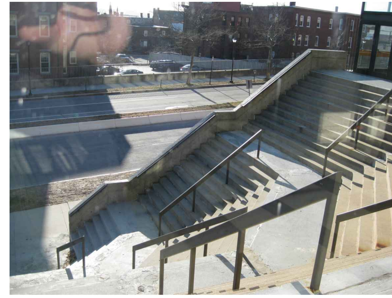
N10 SITE PHOTO
