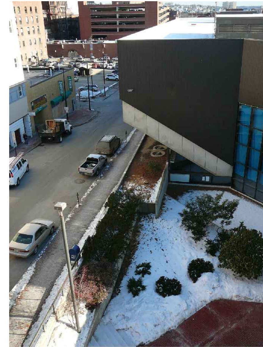
N14 SITE PHOTO
