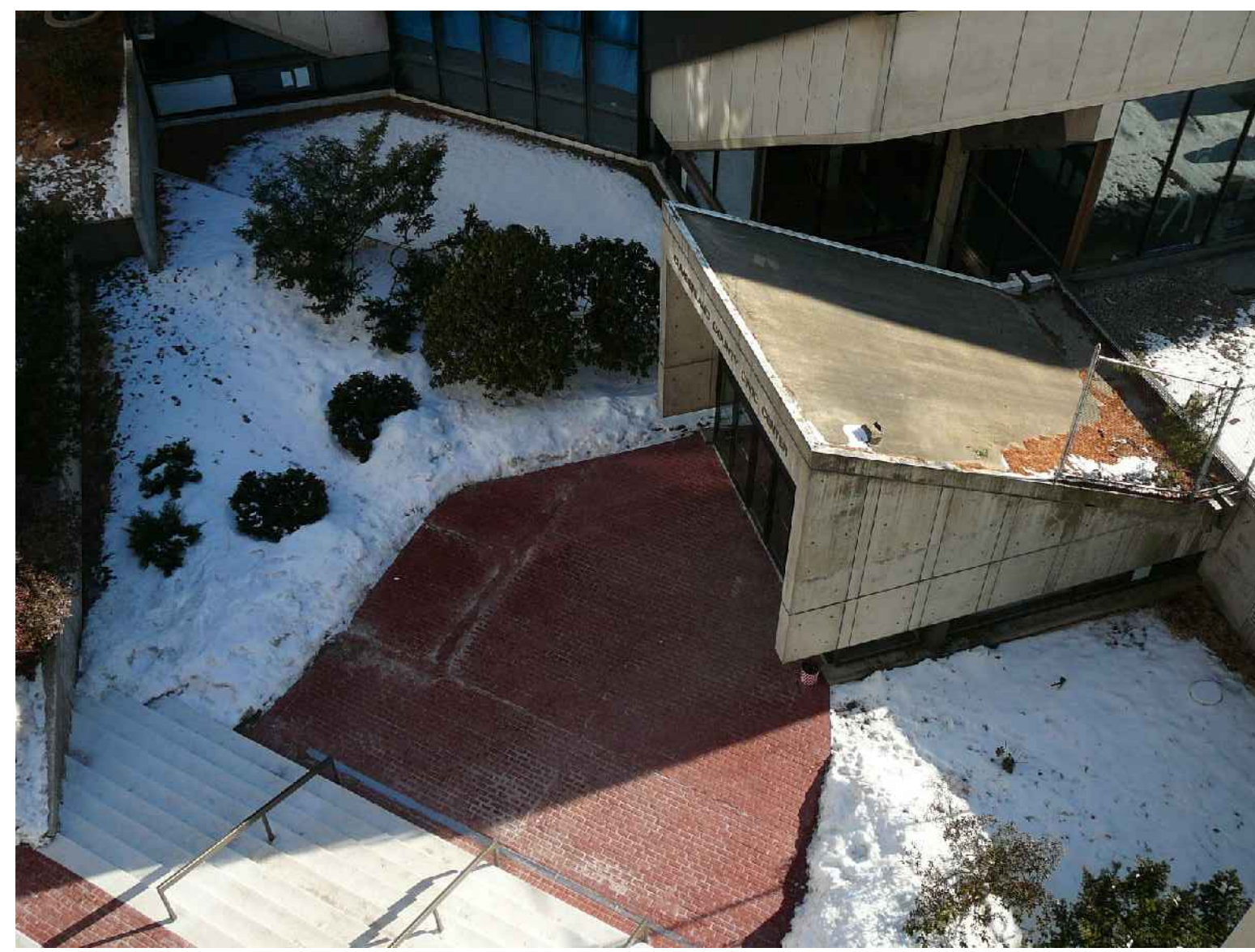
N1 SITE PHOTO
