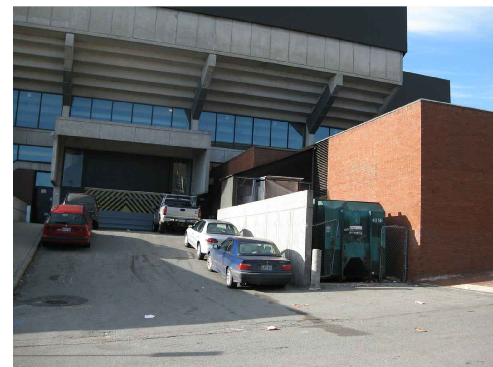
N14 SITE PHOTO
