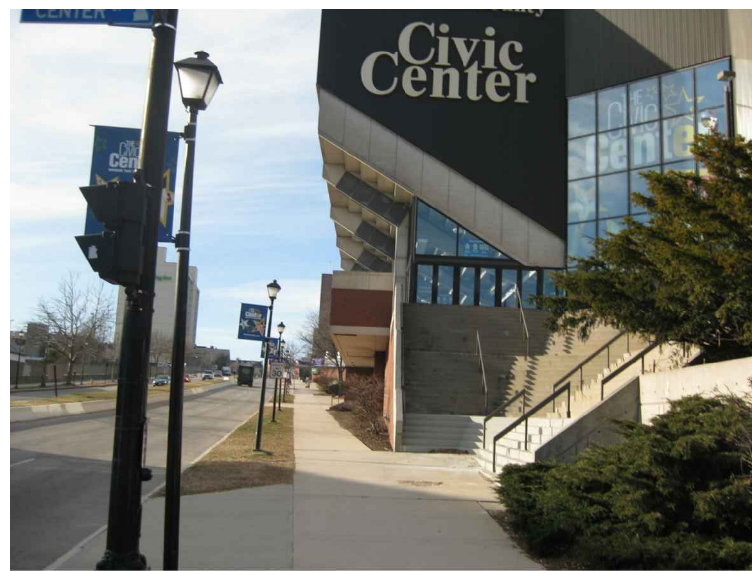
N5 SITE PHOTO
