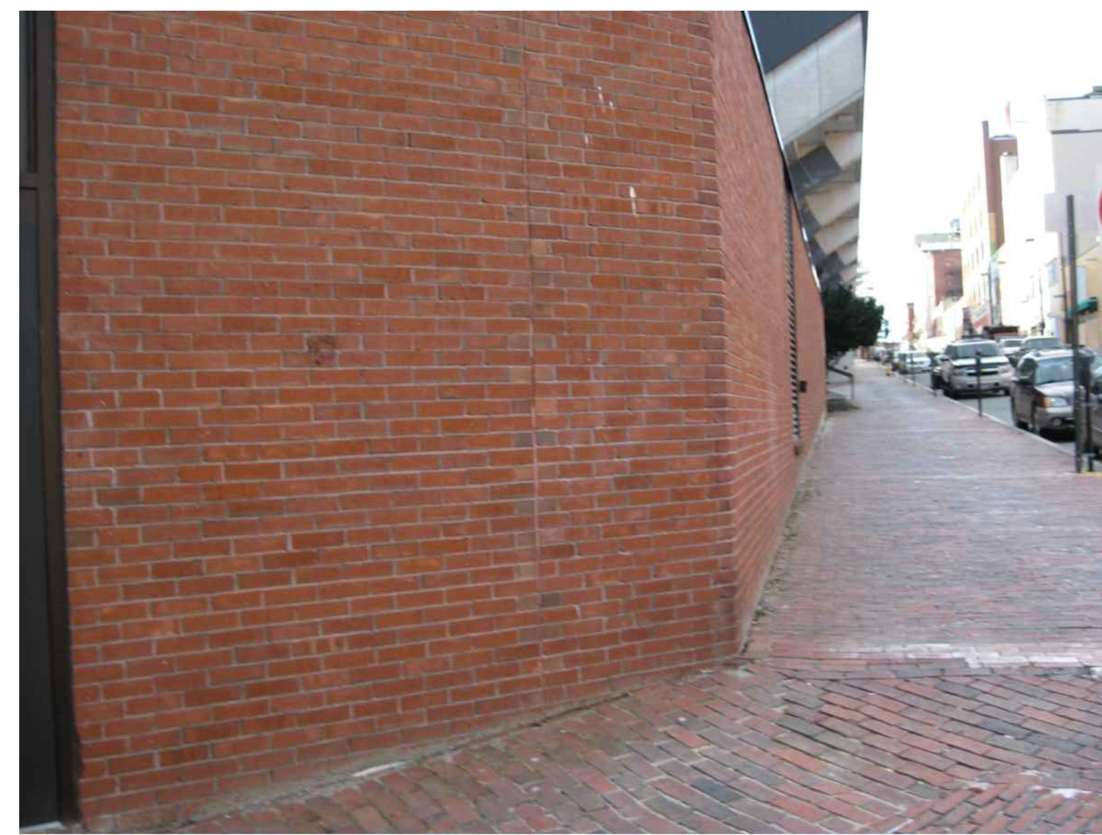
N5 SITE PHOTO
