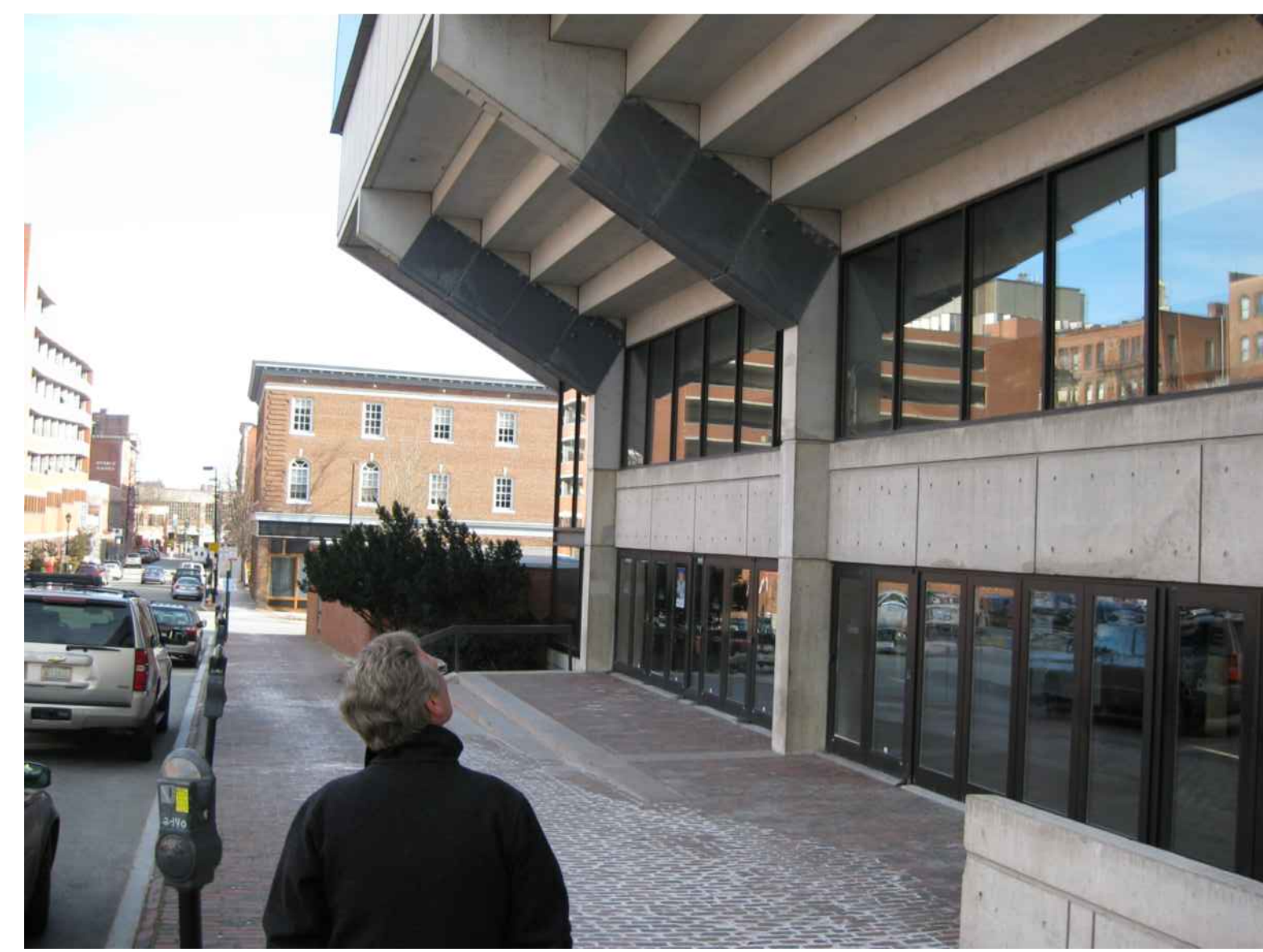
N5 SITE PHOTO
