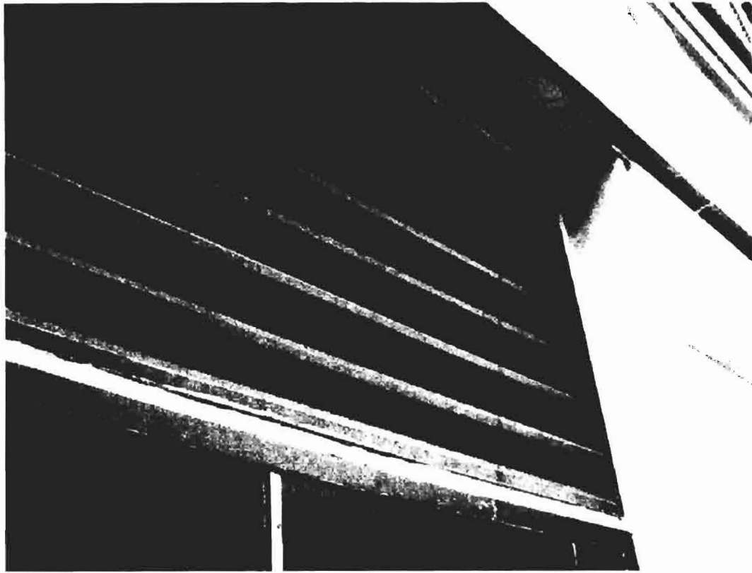
EXTERIOR EXISTING FIXED LOUVER
