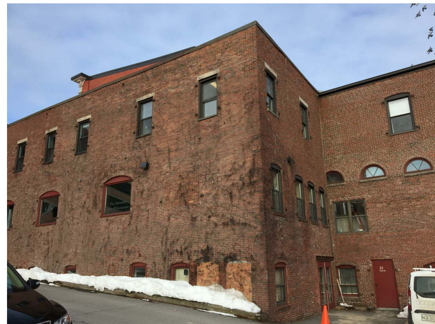
WEST & SOUTH ELEVATION - FROM PARKING LOT
