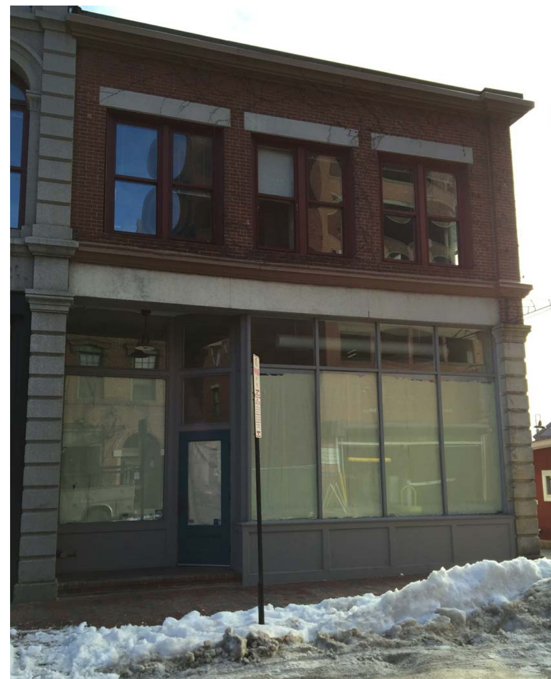
NORTH ELEVATION - FROM FREE STREET
