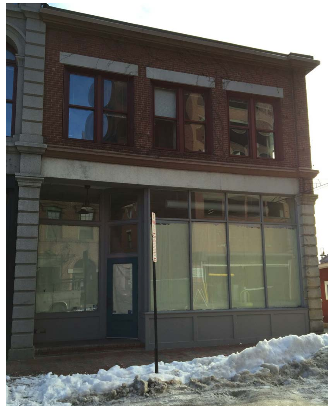
NORTH ELEVATION - FROM FREE STREET
