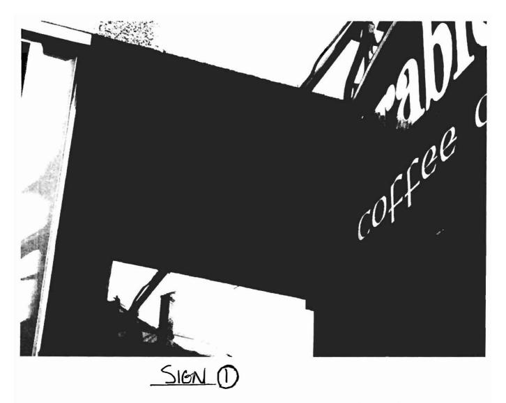
· EXISTING BRACKET TO BE REFUEBBILLED AND RELOCATED WITH SIGN to NEW LOCATION.
