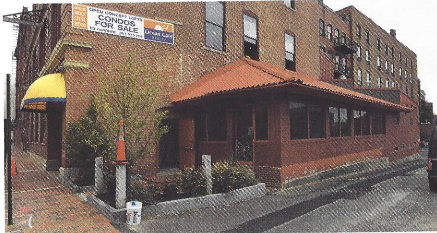
3 EXISTING CORNER VIEW
