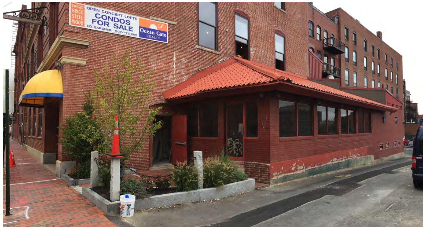
③ EXISTING CORNER VIEW
