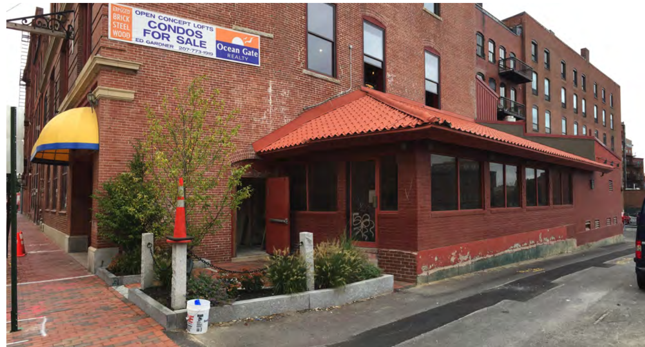
③ EXISTING CORNER VIEW
