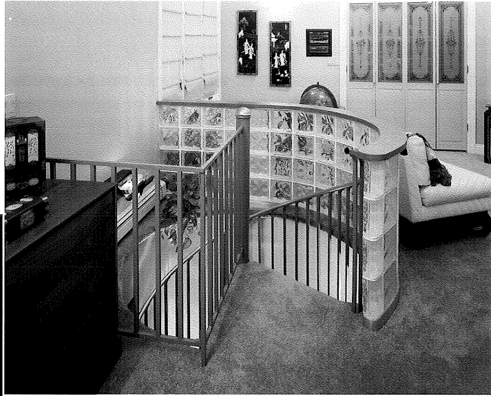
(Left) View from upper level showing optional dome center pole cap and well railing.
