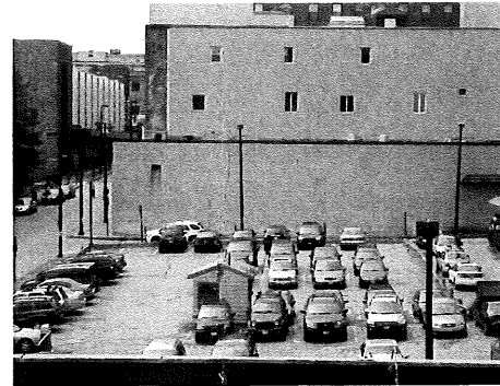
6 View from Monument Square Parking Garage NTS
